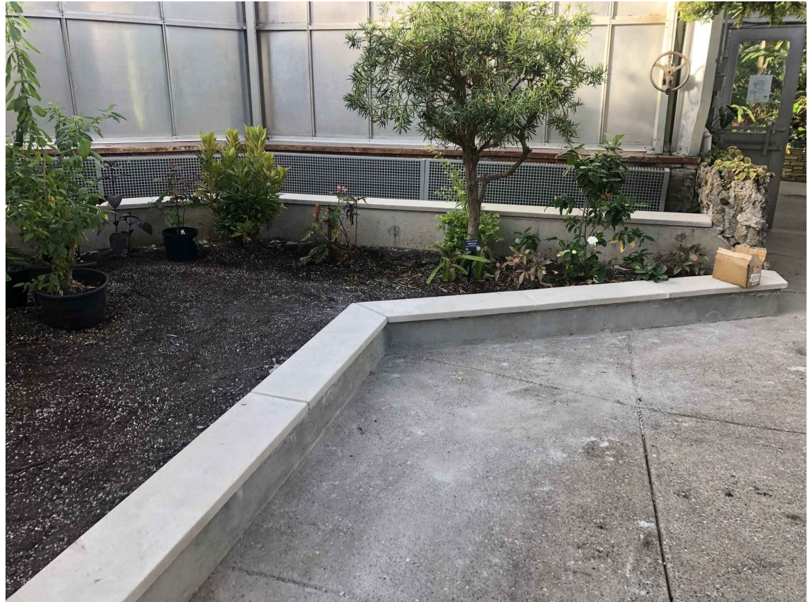
Limestone cap installation in showroom underway.
