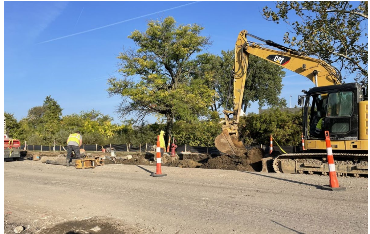
Excavation for one of two hydrants along Riverbank.
