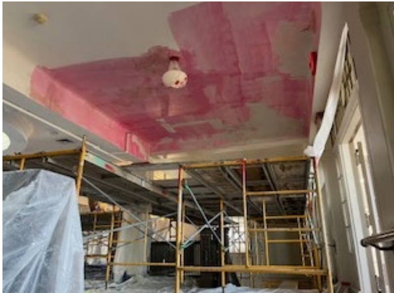
Interior plaster repairs at the Casino.
