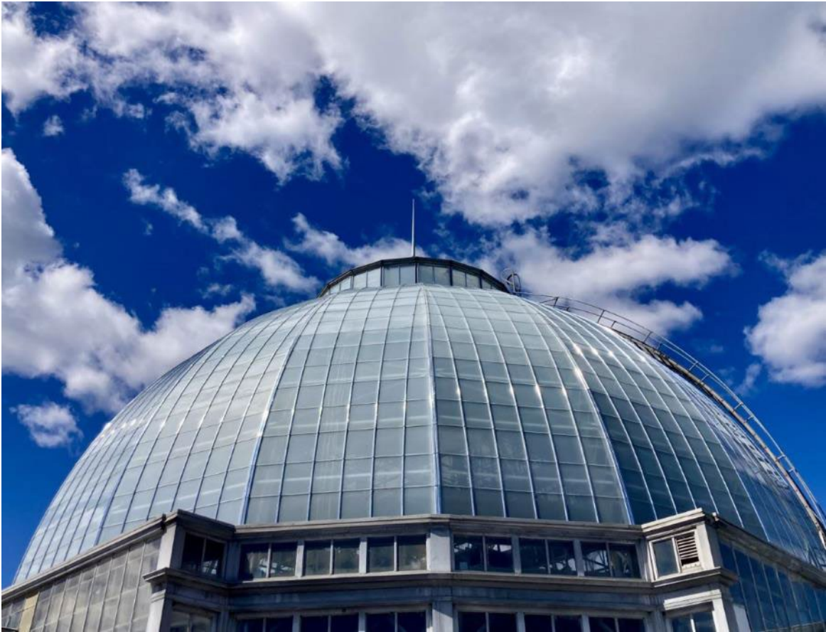
Abatement, steel repairs and new paint followed by reglazing were key items addressed.
