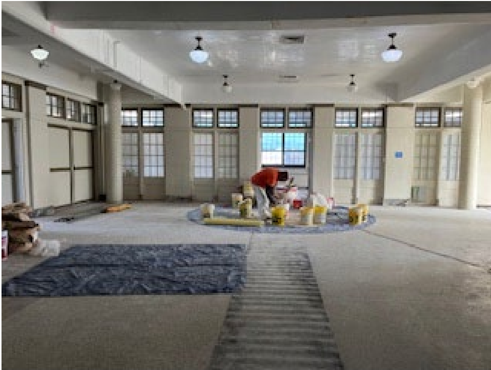
Significant plaster repairs need from the leaking roof before repairs on second floor.
