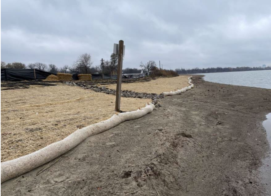
Belle Isle sourced plantings installed along the Wilson Trail.
