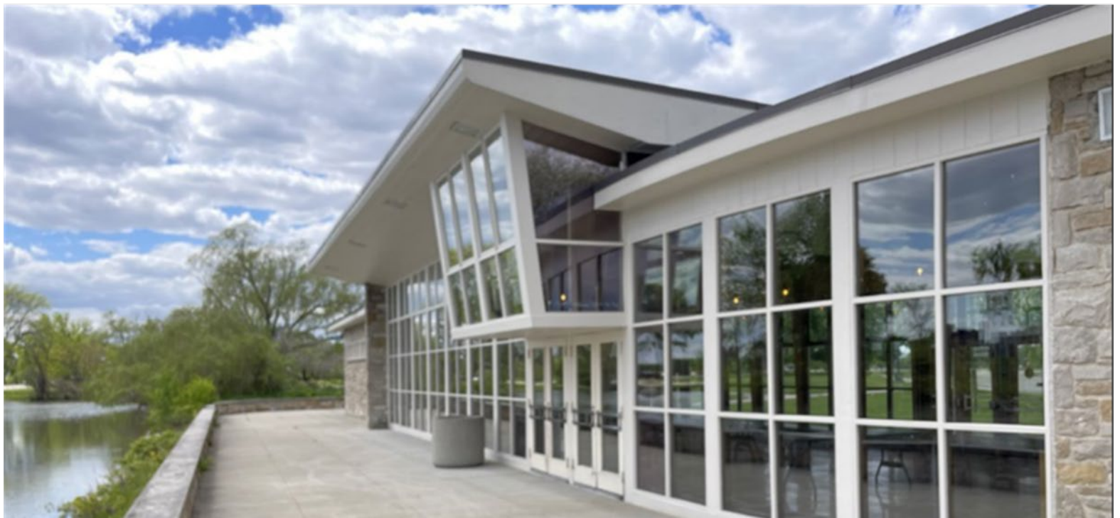
Significant repairs to replace deteriorated wood framing.
