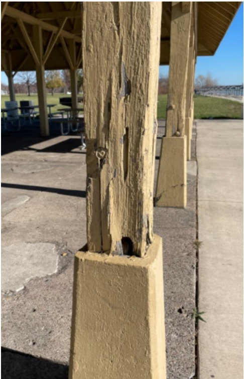
Parkwide structure review identified structural repairs required at Shelter #9
