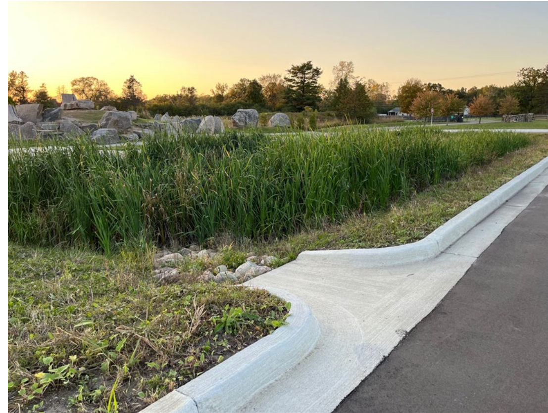
GEI parking lot example providing stormwater management and habitat, Carpenter Lake, Southfield, MI.
