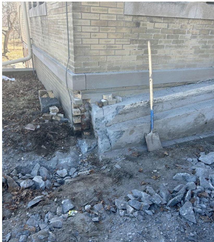
Intended removal of cheekwall review, wall was poured up against brick wall.
