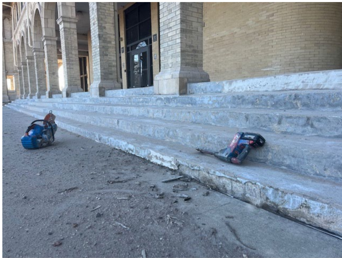
Removing delaminated surfacing from steps and porch.
