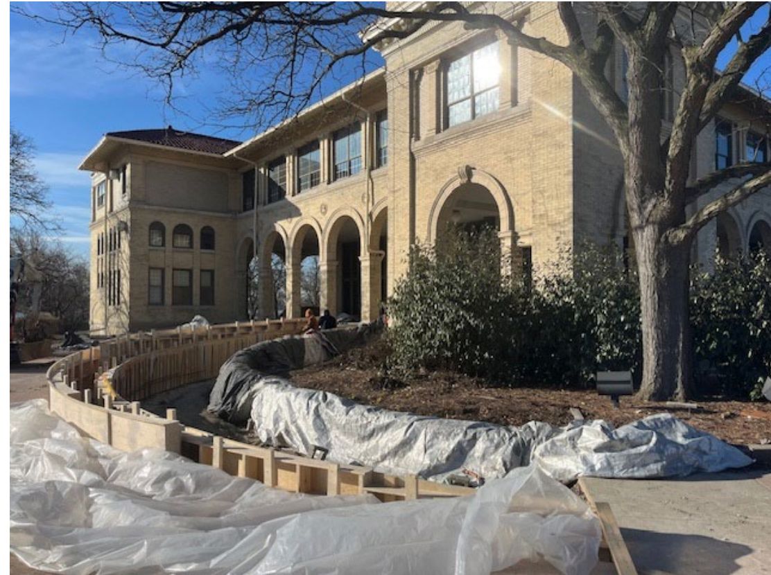
Covering new concrete during cold temperatures.
