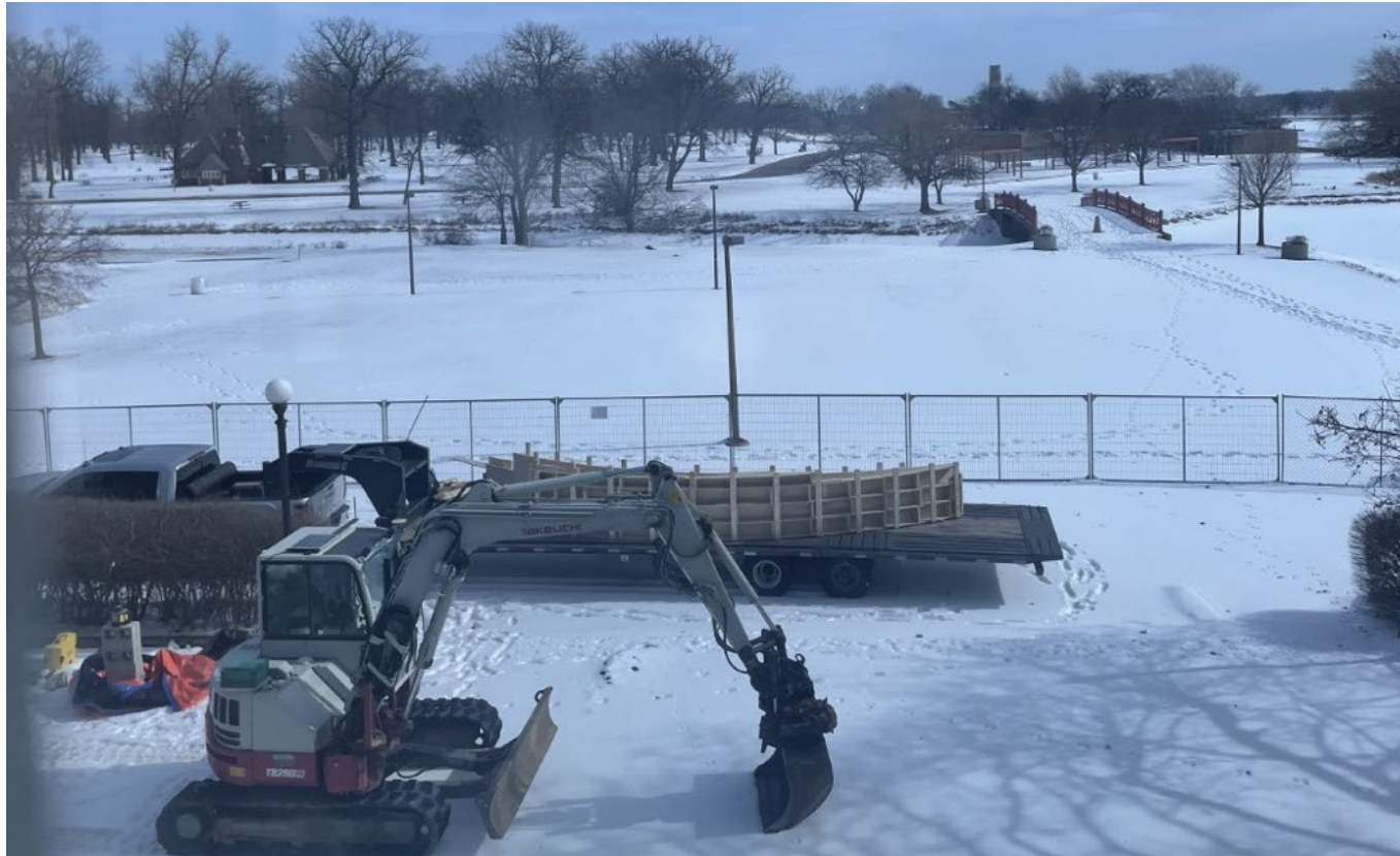
New ADA accessible walk formwork constructed off site and brought to park.
