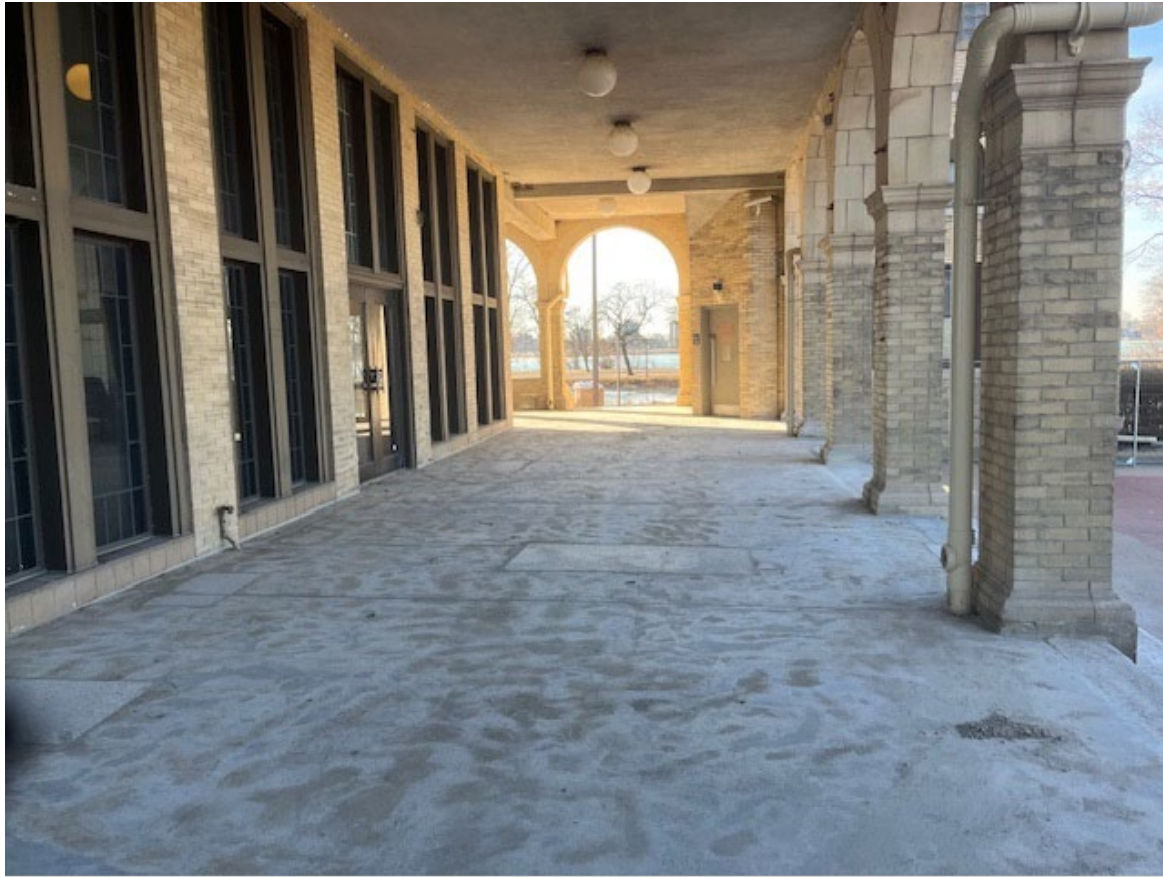
Removal of deteriorated and delaminated surfacing around porch.
