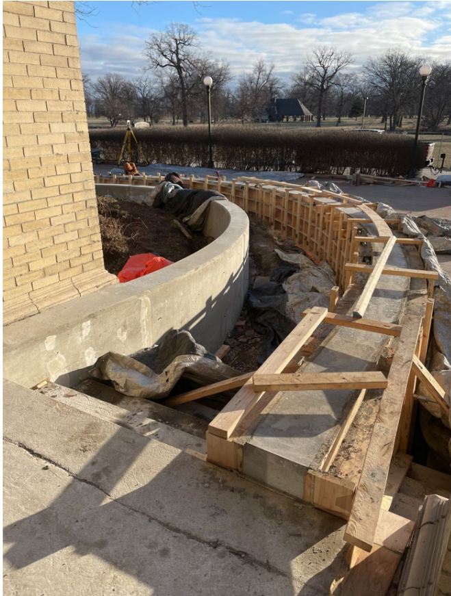
New ADA accessible walk formwork
