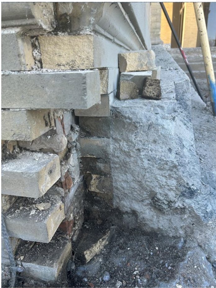
Intended removal of cheekwall review, wall was poured up against brick wall.
