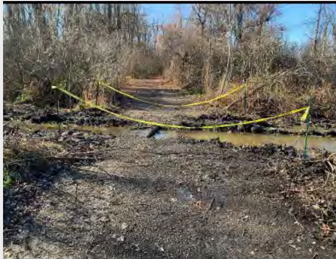
1) Oakway ditch #1 installed across walking path
