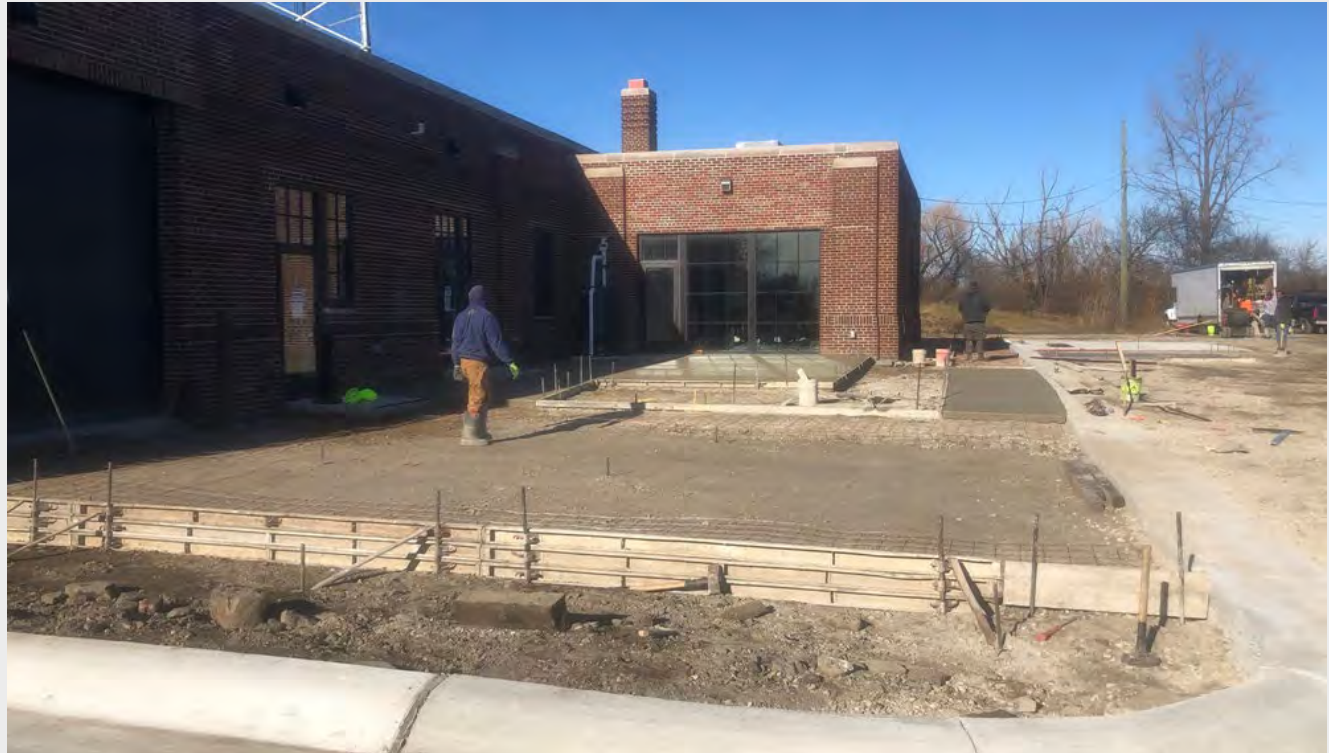
ADA access and paving scheduled for Park HQ
