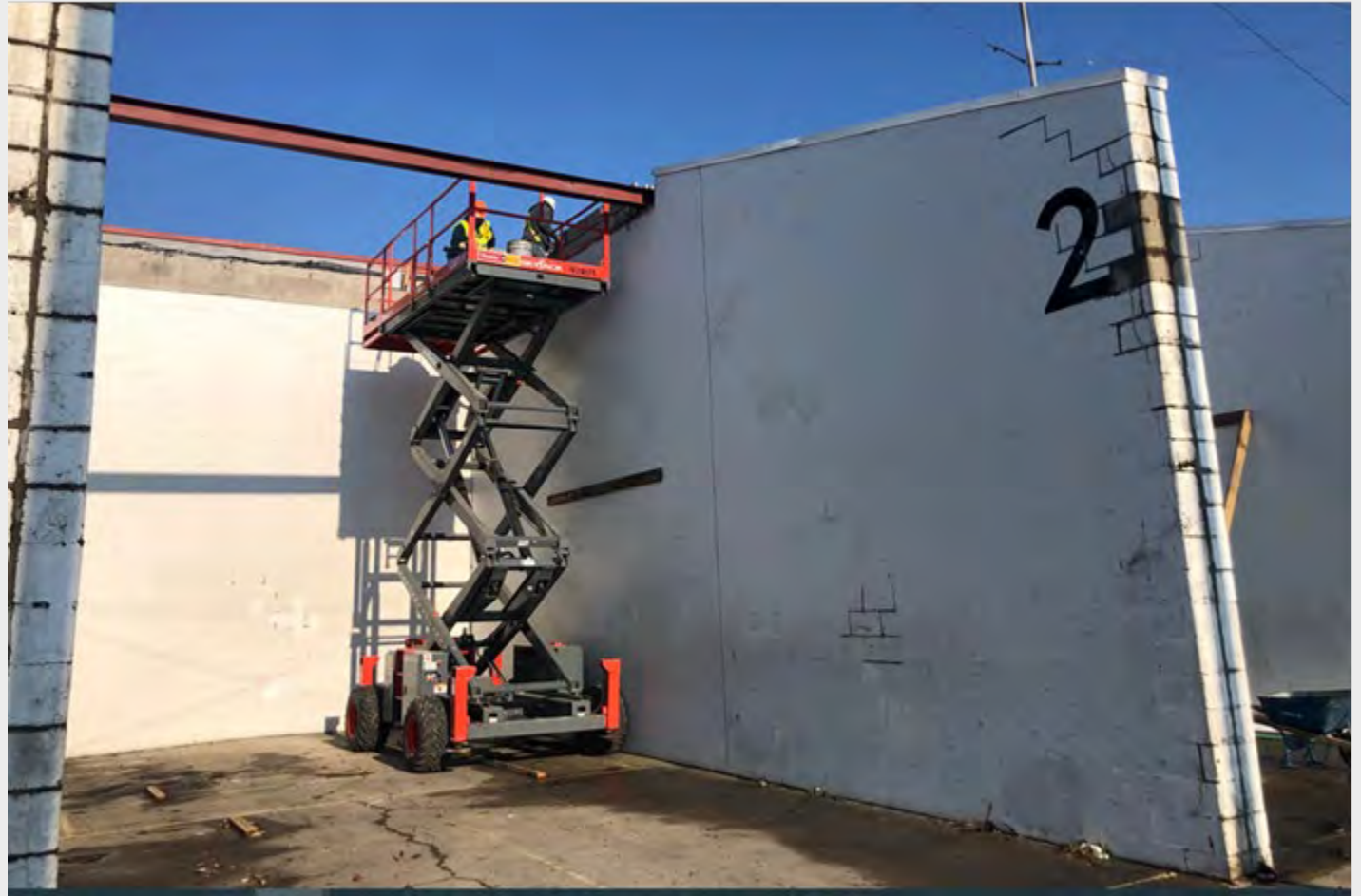
Additional Masonry work required once roof structure was removed
