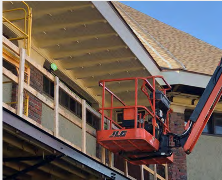
New painted soffit and supports being installed
