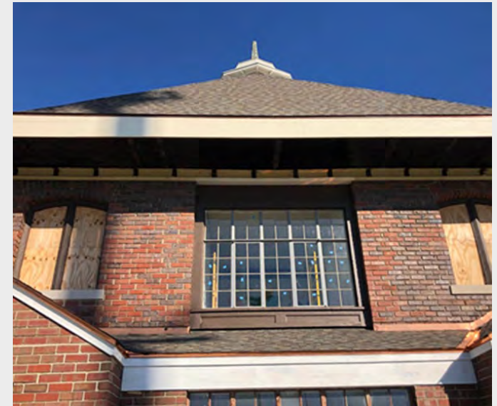
Newly painted window and fascia
