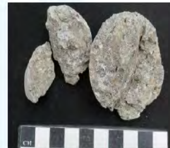
PHOTO NO. 7B: Core No. 2 – Loose/fractured fragments of original concrete at the base of core.
