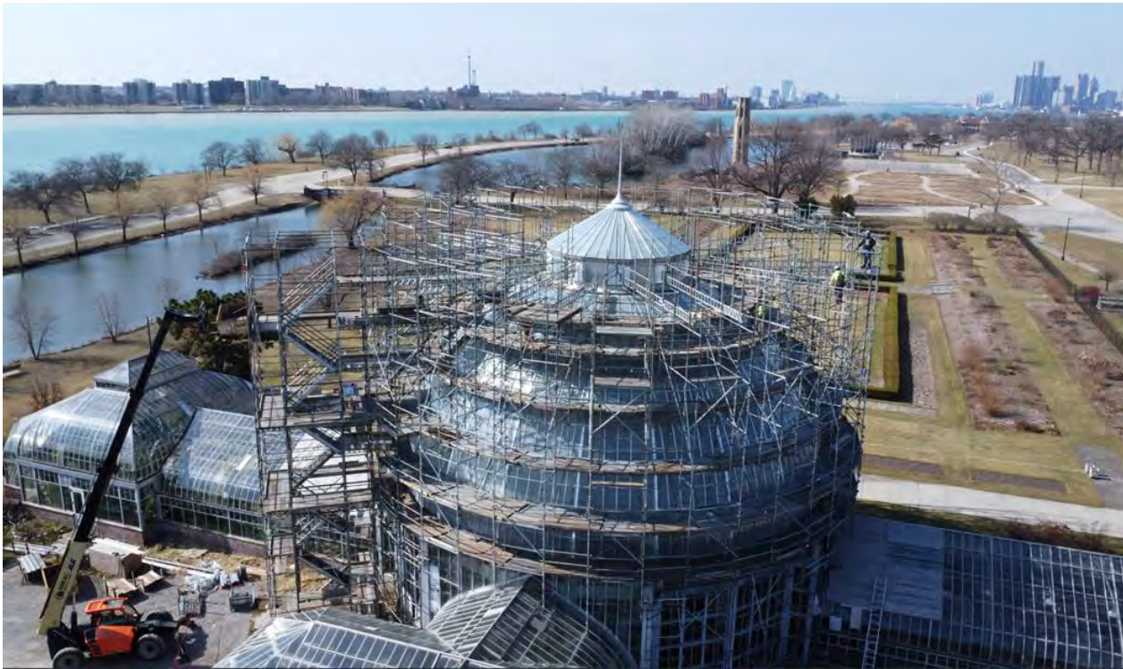
Conservatory dome glass replacement complete and scaffolding removal underway.
