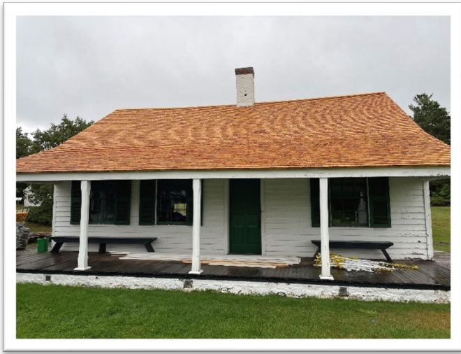
Fort Wilkins Historic Complex Hospital Building Re-Shingling
