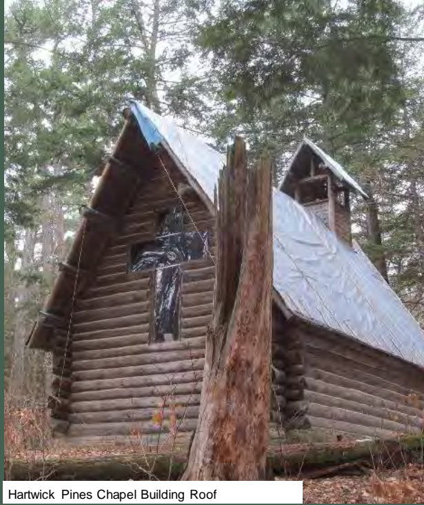
Hartwick Pines Chapel Building Roof
