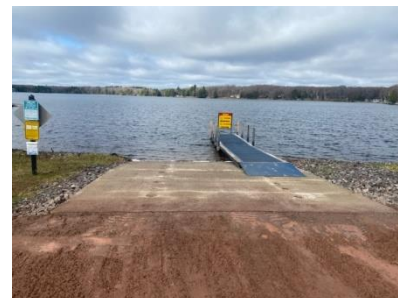
REPAIRED RAMP AT CISCO LAKE BAS IN GOGEBIC COUNTY
