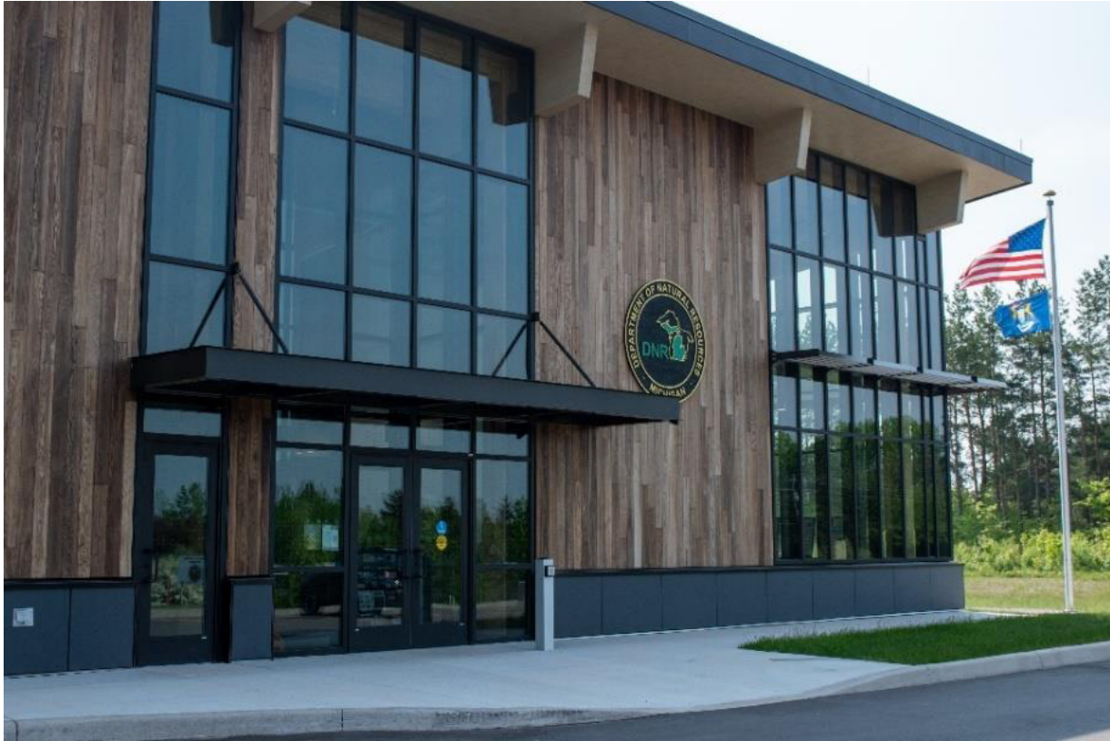
Figure 7. The DNR's new Customer Service Center in Newberry, Michigan, was built using mass timber materials made in part from Michigan-harvested wood.
