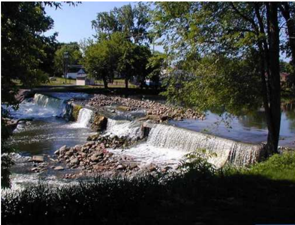
Chesaning Dam breached 2005
