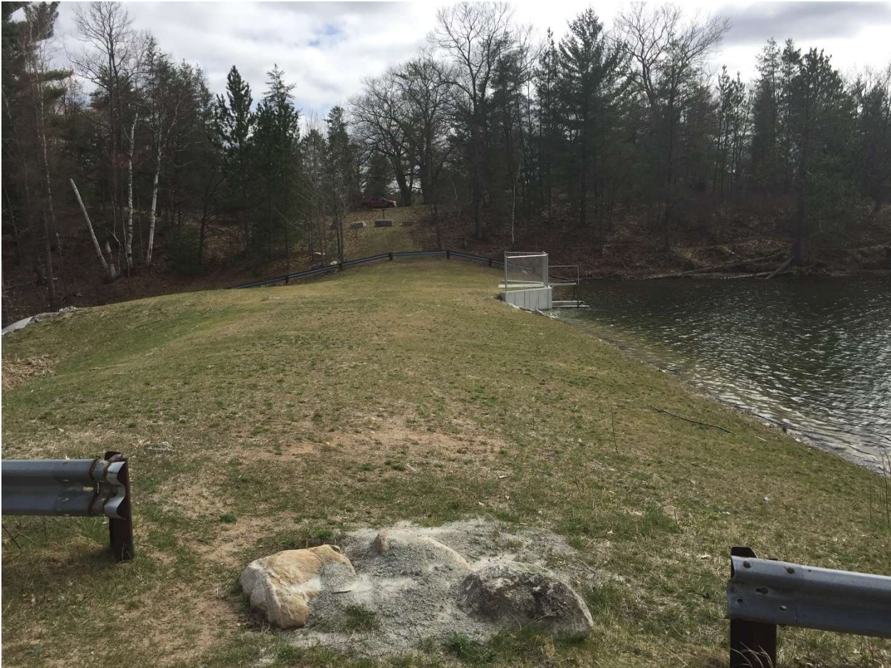
Photo 4. Foch Dam control structure and levee post renovation 2016.
