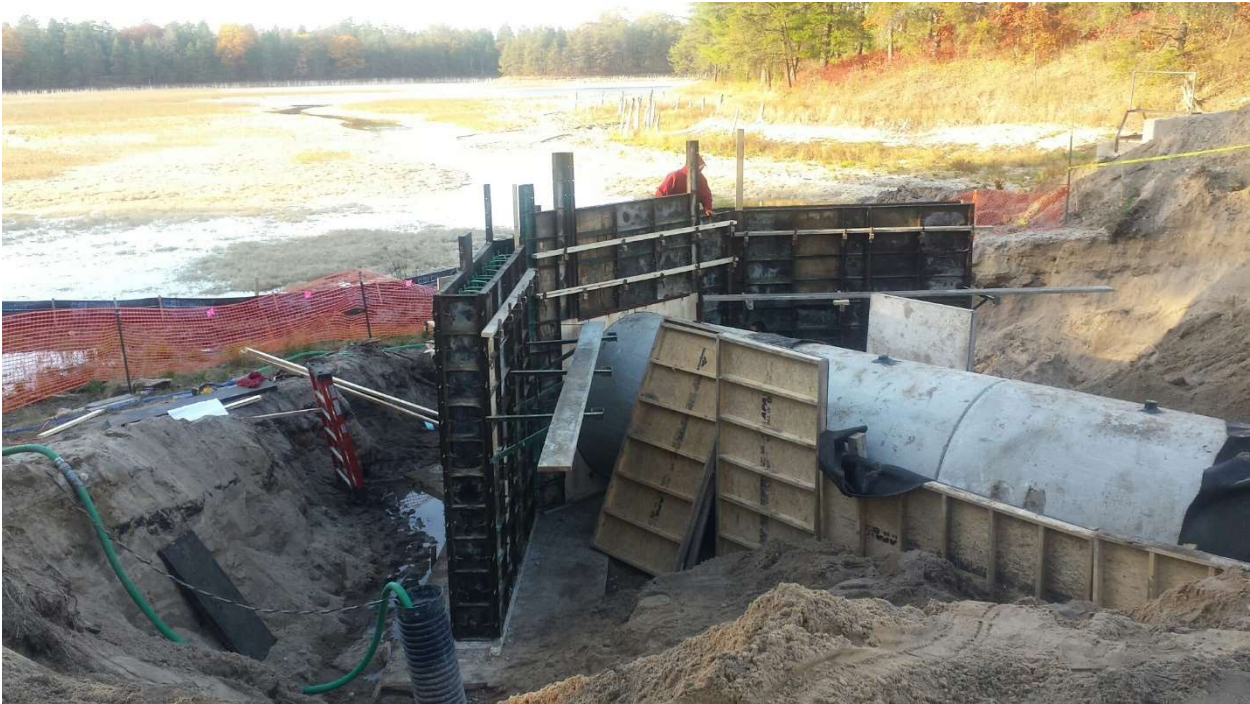
Photo 3. Foch Dam control structure under renovation in 2016.
