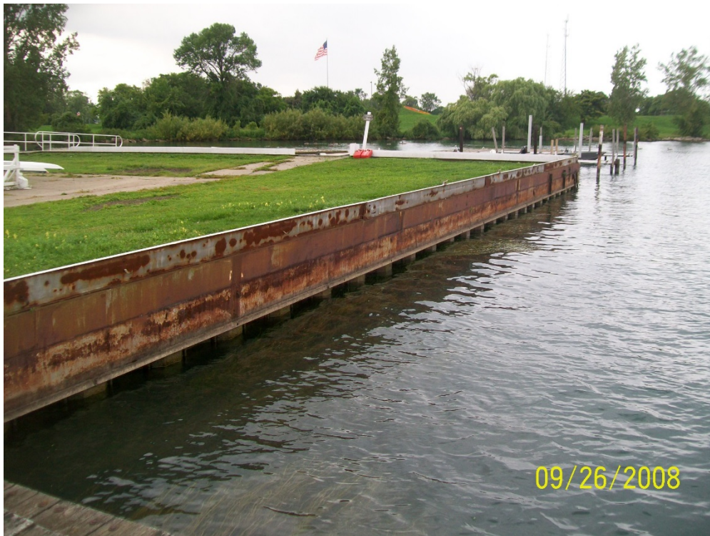
Typical Sheet Pile Wall along North Side of Island (Looking West from T-Pier)
