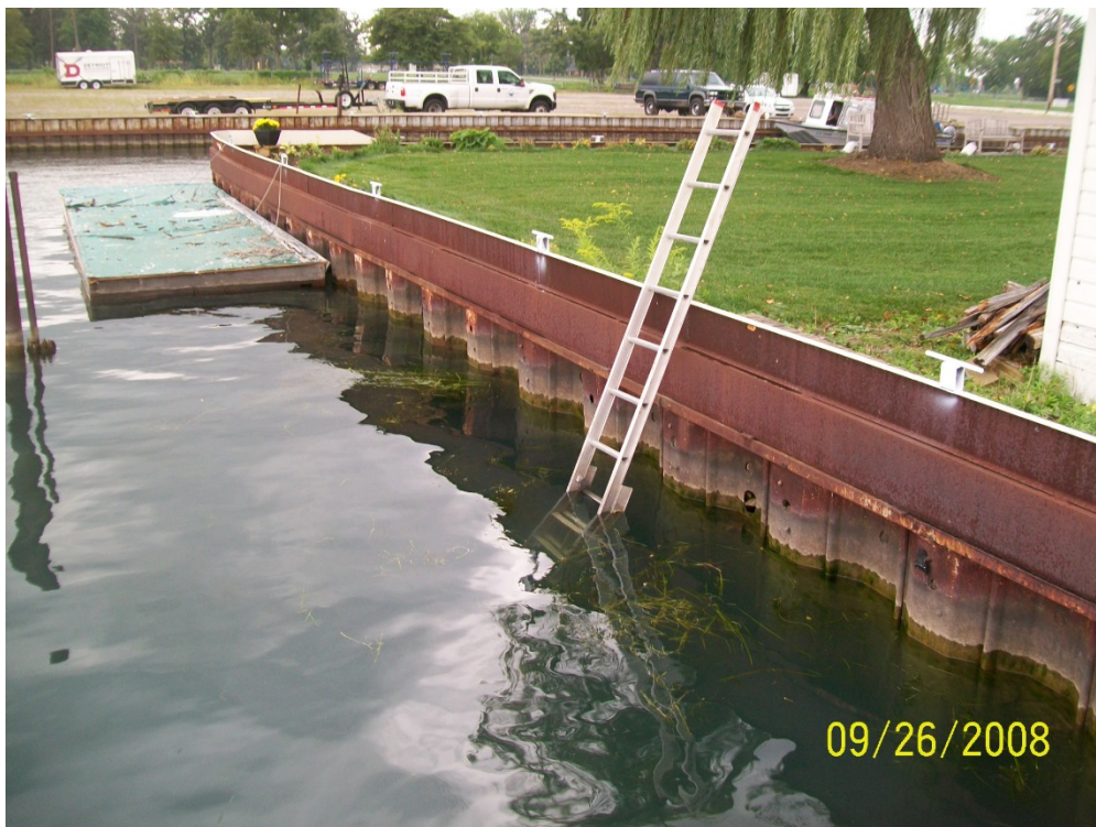
Typical Sheet Pile Wall along East Side of Island (Looking Southwest)
