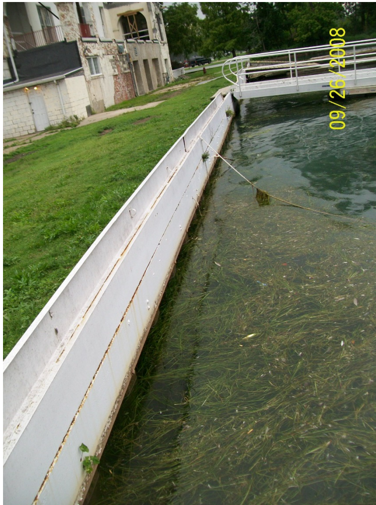
Typical Sheet Pile Wall along West Side of Island (Looking South)
