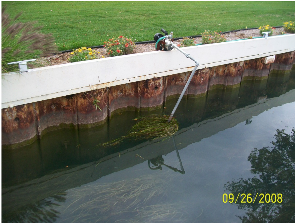
Typical Sheet Pile Wall along South Side of Island (Looking North)
