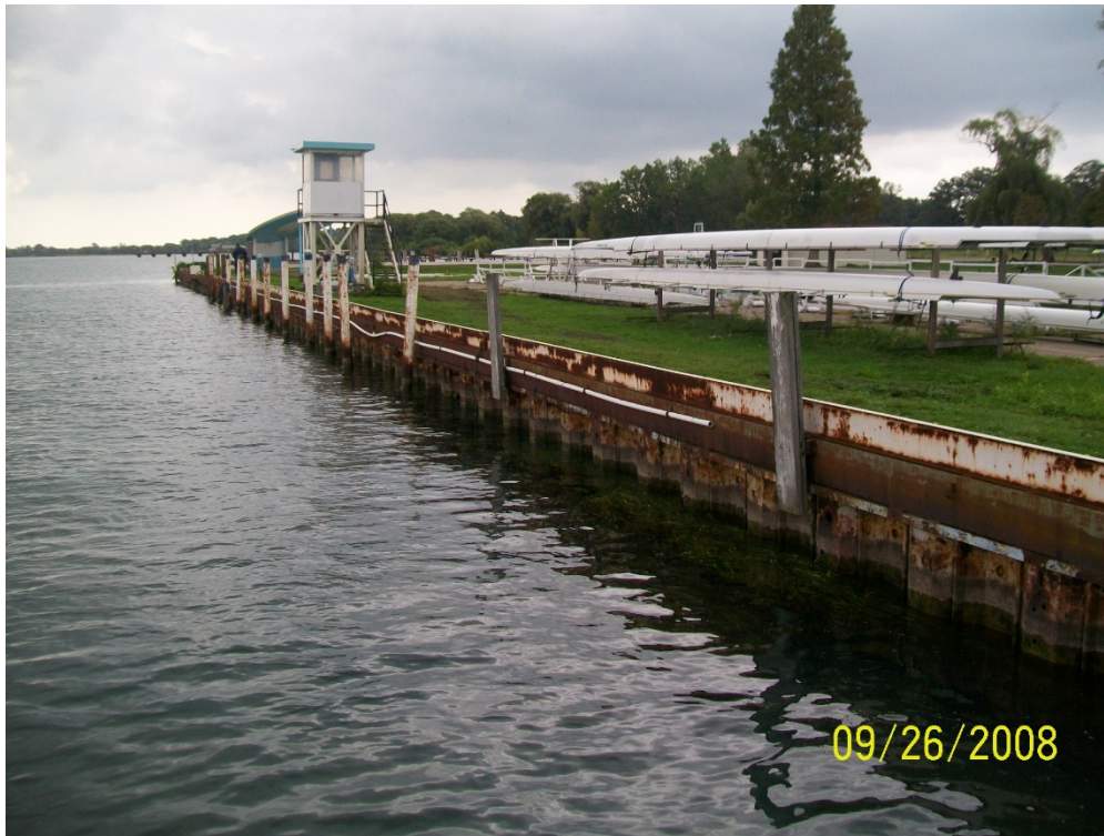
Typical Sheet Pile Wall along North Side of Island (Looking East from T-Pier)
