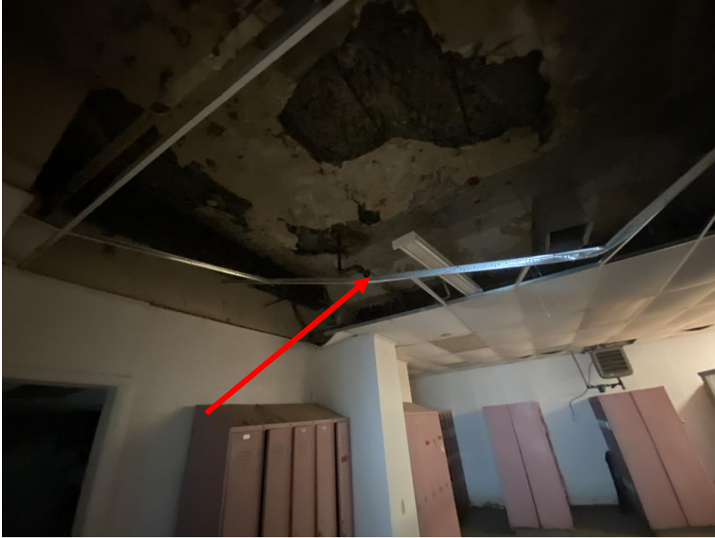
Exposed Pipe Insulation
