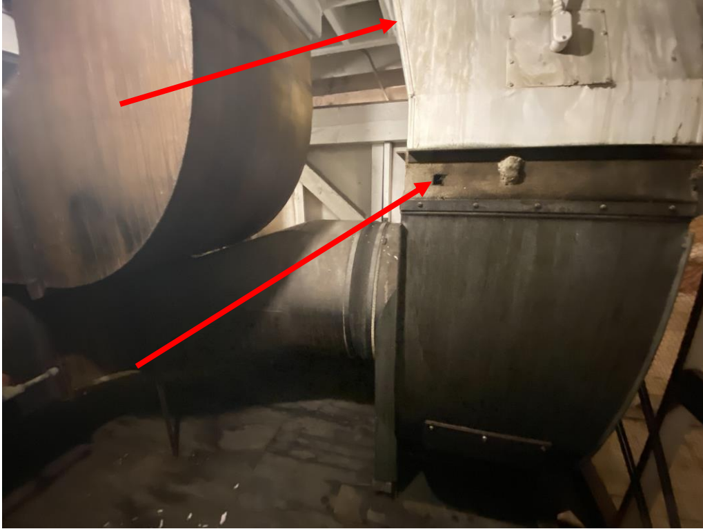
Vibration Dampener and Duct Wrap (HA 74 & HA 113)
