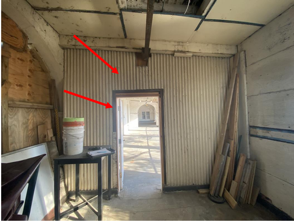
Transite Panels and Interior Caulk (HA 104 & H A112)
