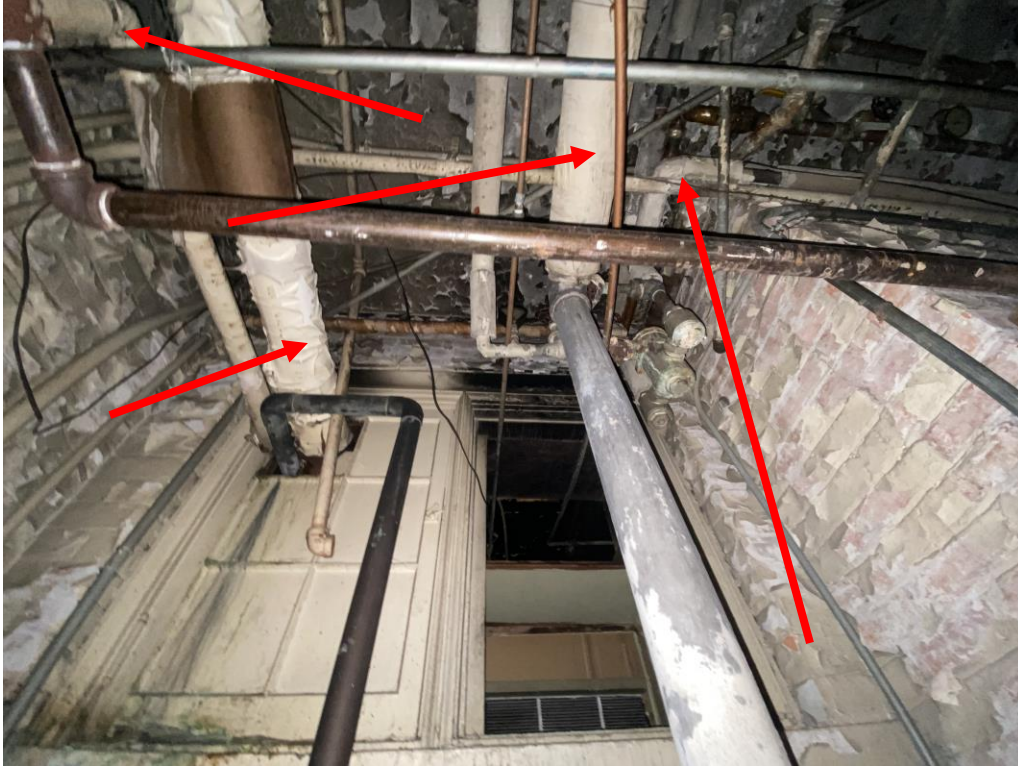
Pipe Insulations and Pipe Fittings (HA 69, 70, 71 & 72)
