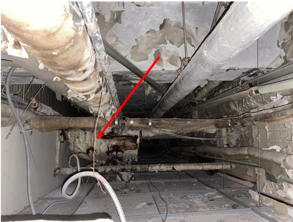
Severe ACM Damage
