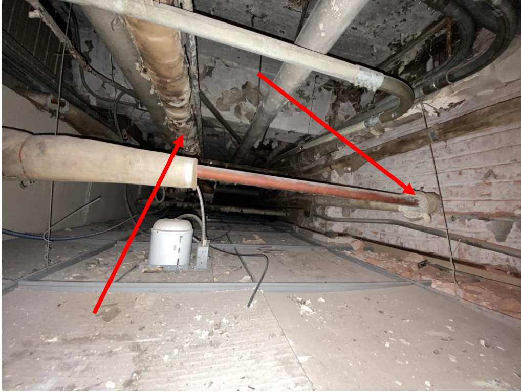
Severe ACM Damage
