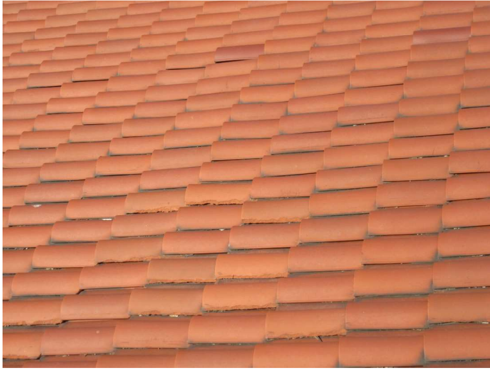
Photo 45 Damaged Spanish Tiles
