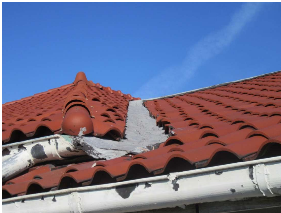
Photo 48 Mastic Over Valley Flashing
