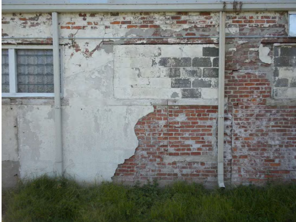
Photo 6 Spalled Stucco
