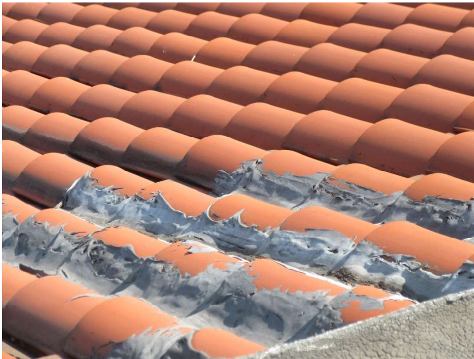
Photo 46 Roof Mastic Repair
