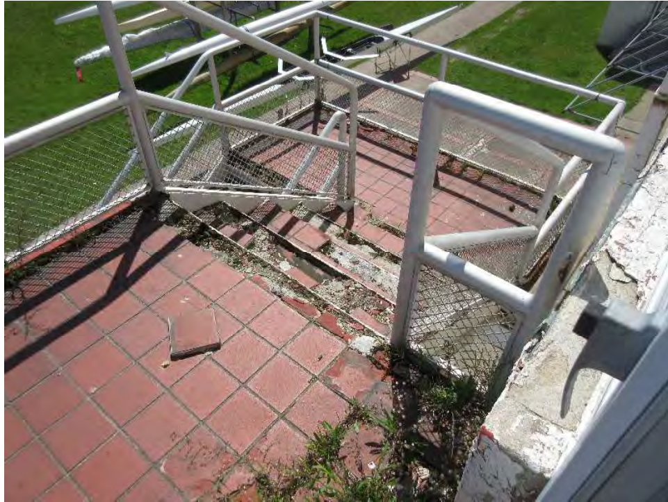
Photo 27 Northeast Staircase Deteriorated Treads
