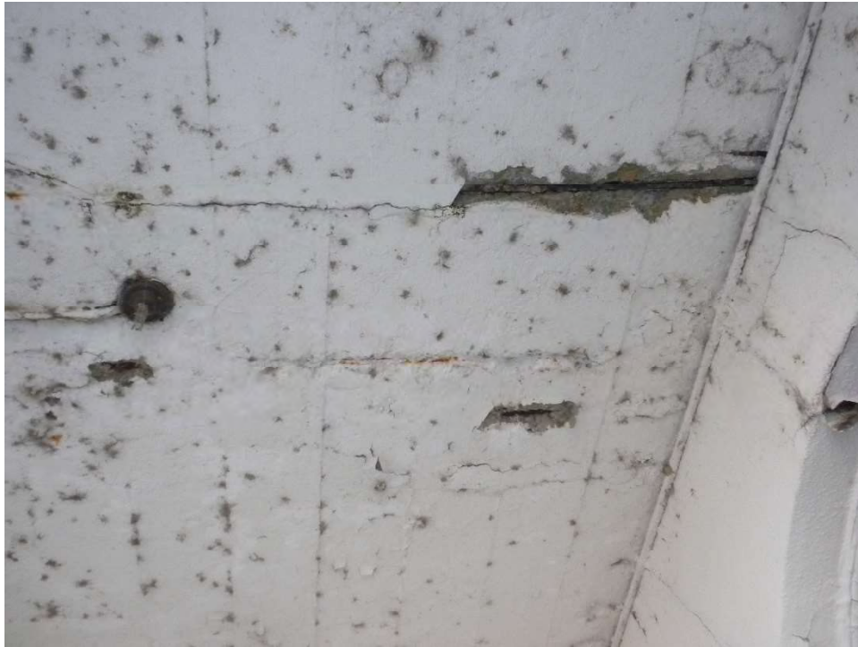
Photo 15 Damaged Stucco – Surface Scaled Finish
