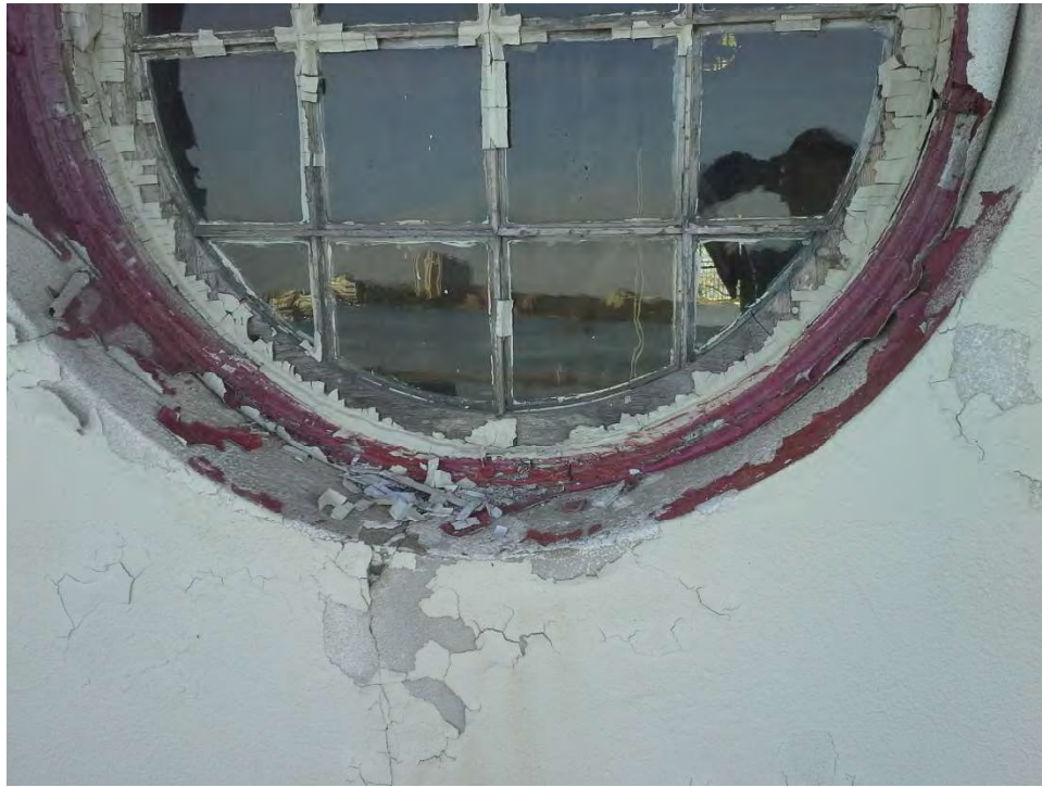
Photo 39 Deteriorated Paint and Wood
