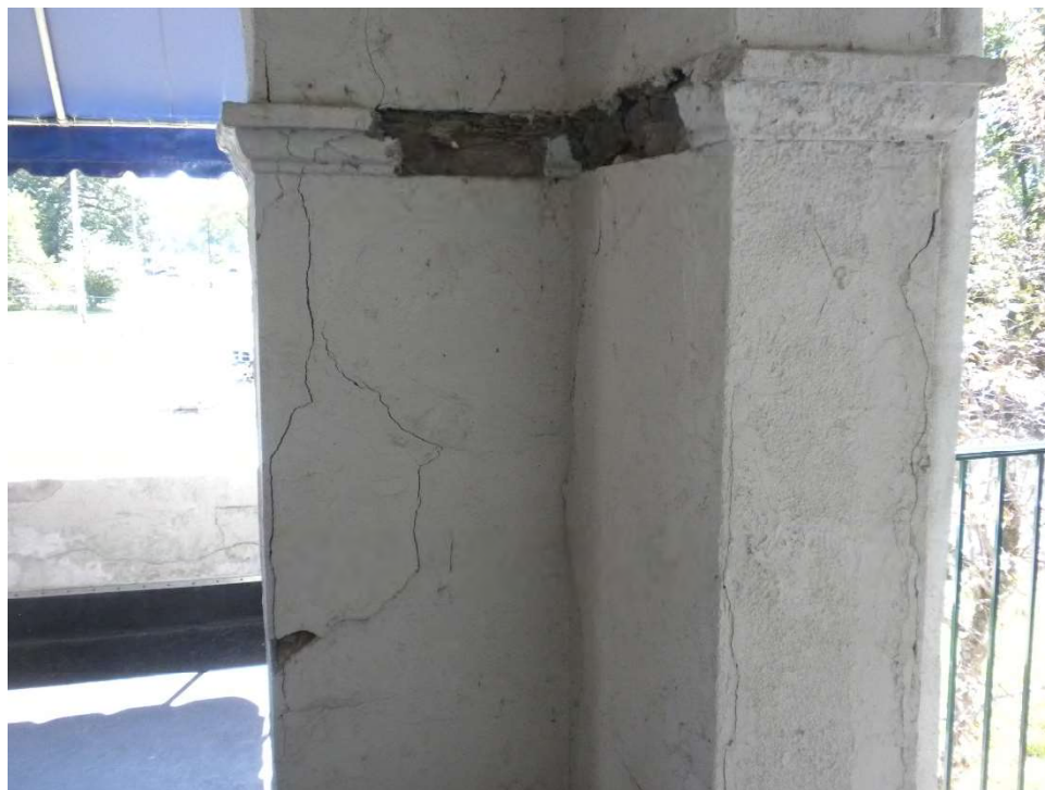
Photo 8 Damaged Stucco – Surface Scaled Finish
