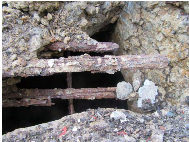
Photo 82 Badly Deteriorated Reinforcing Steel
