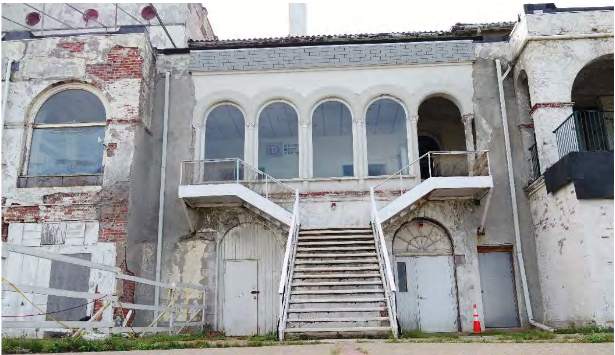
Photo 26 North Staircase Corrosion
