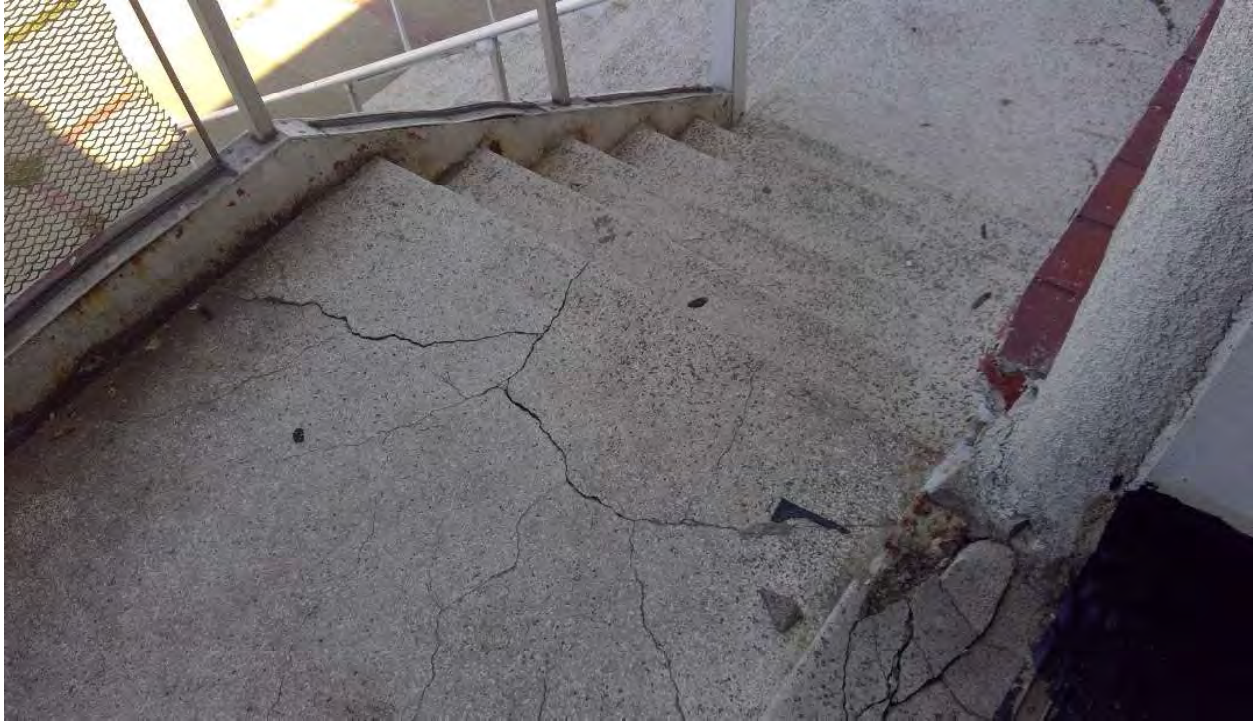
Photo 25 North Staircase Deteriorated Landing
