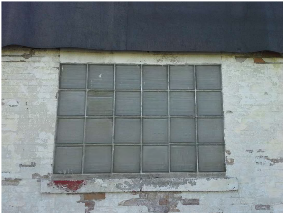
Photo 38 Glass Block Infill
