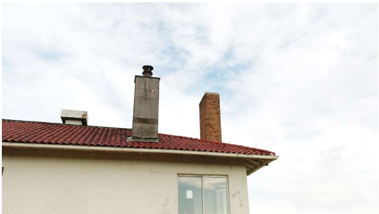
Photo 32 Plywood Clad Chimney
