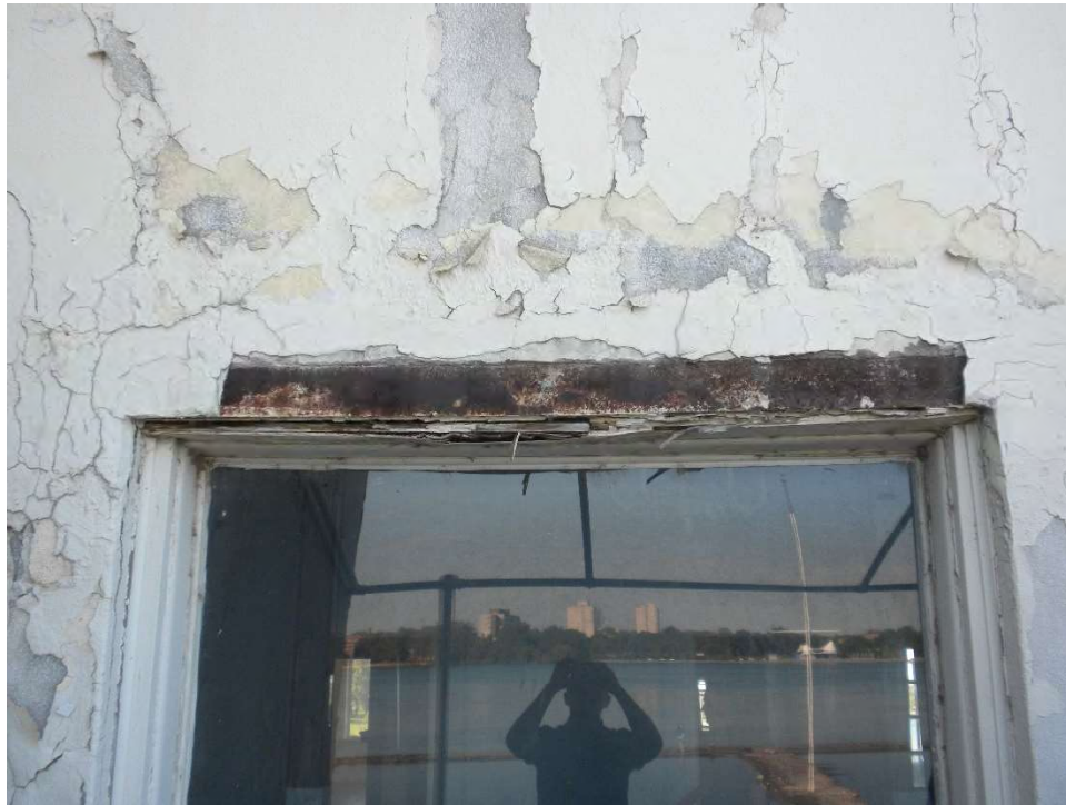
Photo 11 Damaged Lintels
