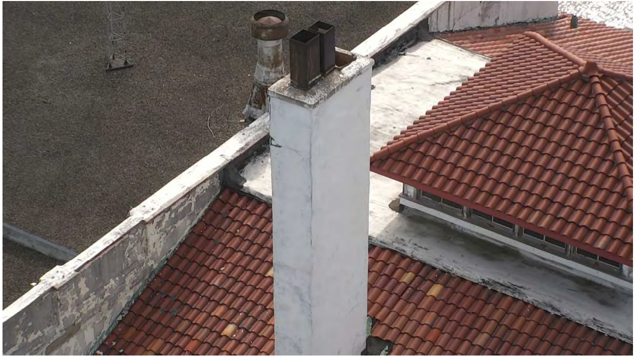
Photo 29 Debonding Stucco on Chimney
