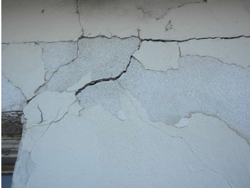
Photo 7 Debonded Stucco (Back-side of covered terraces)
