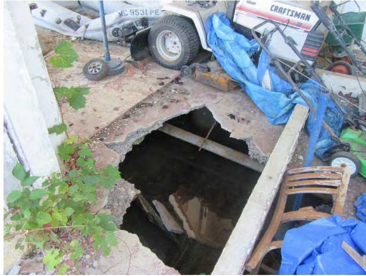
Photo 79 Hole in Pool Deck Below Northeast Terrace 2019
