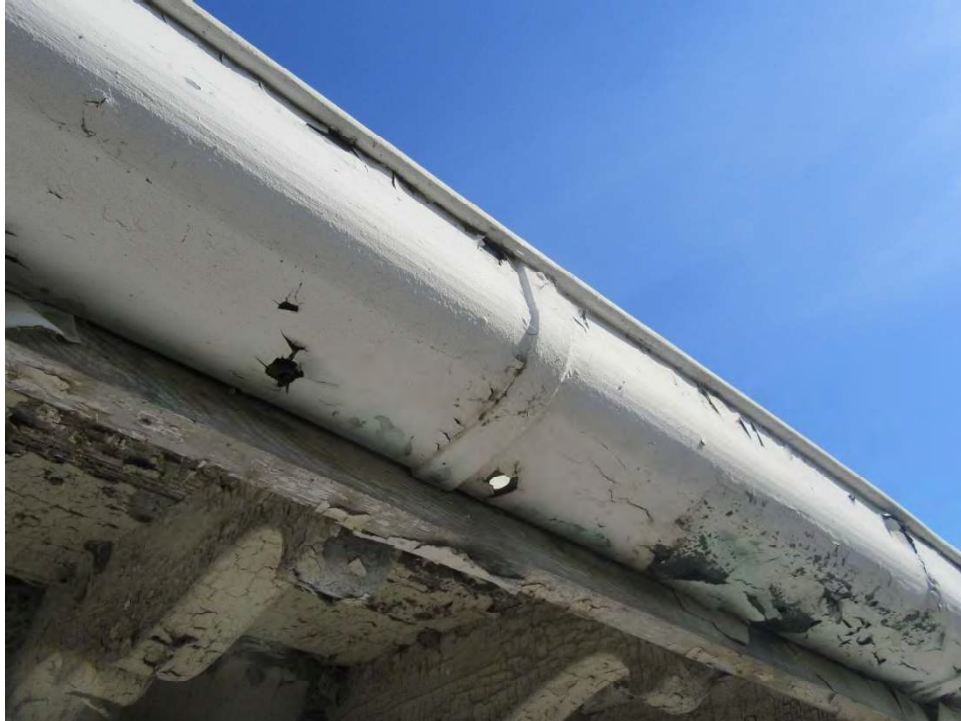
Photo 73 Typical Holes in Gutter
