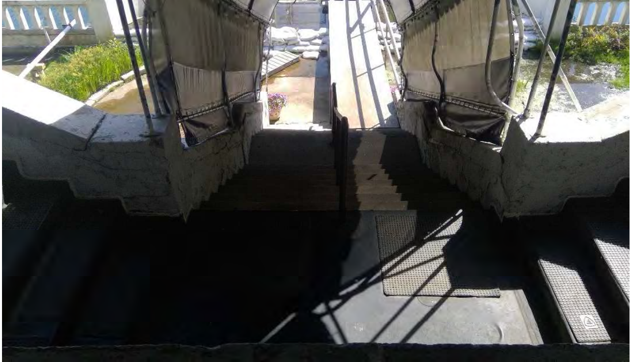
Photo 23 South Staircase Deteriorating Copings
