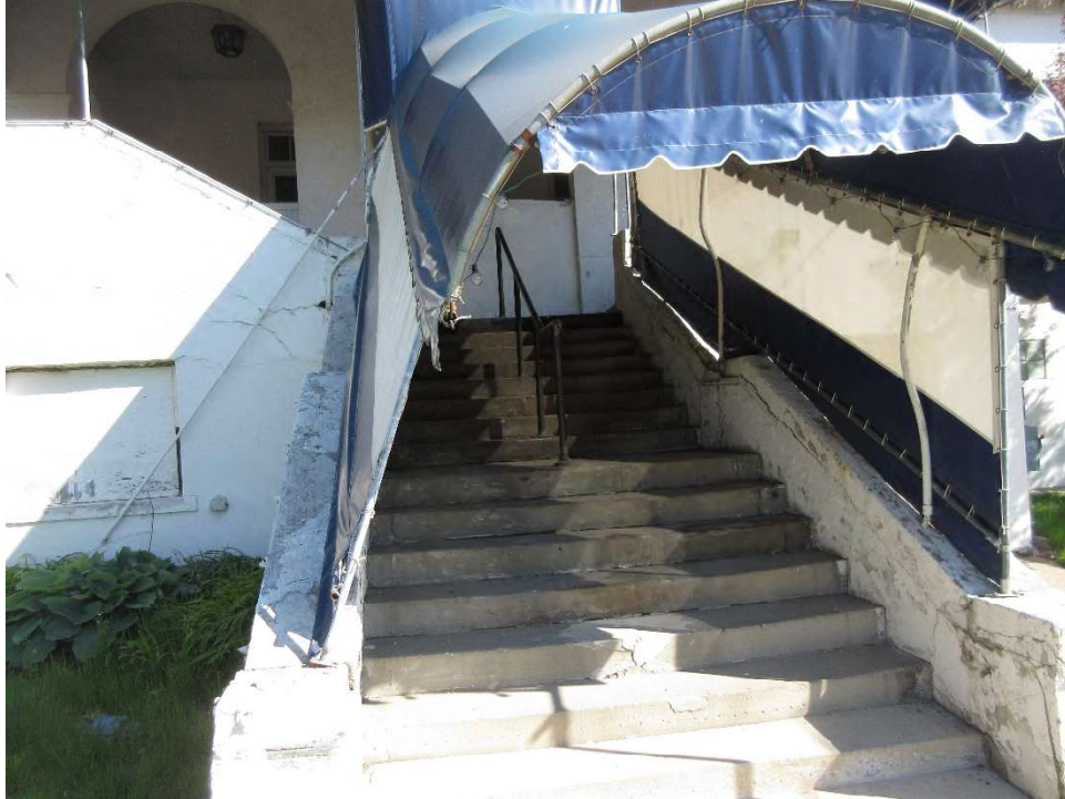
Photo 22 South Staircase Deteriorated Concrete Steps
