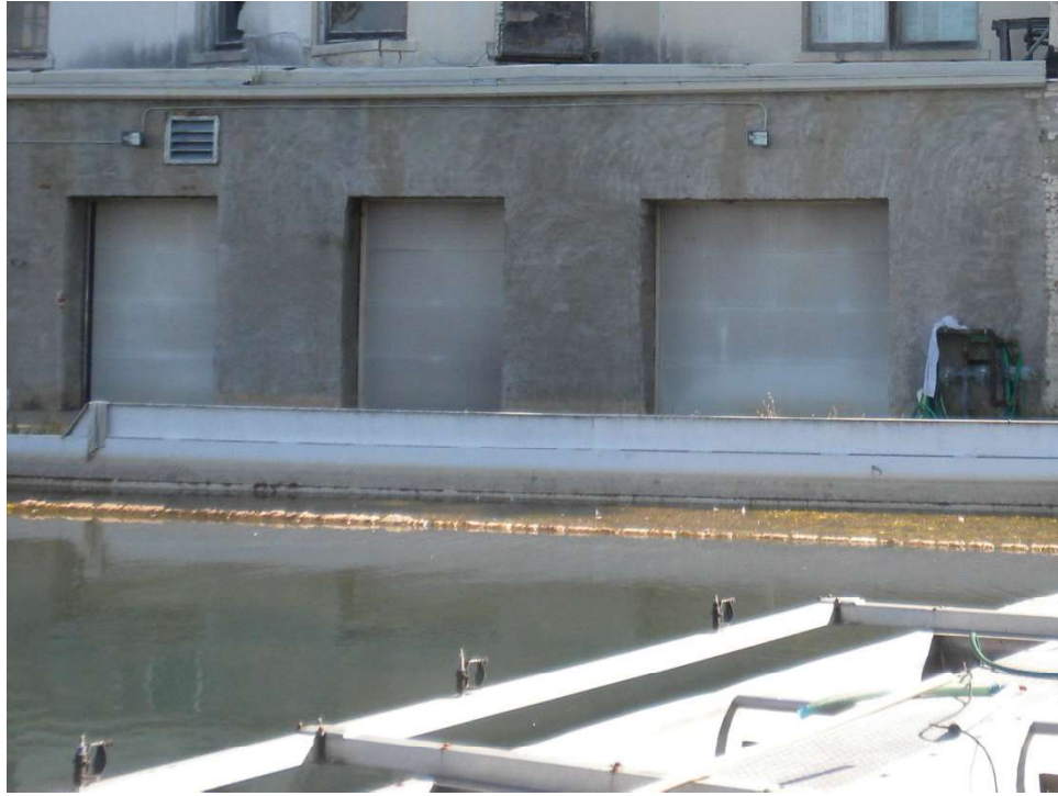
Photo 9 Previously Repaired Stucco
