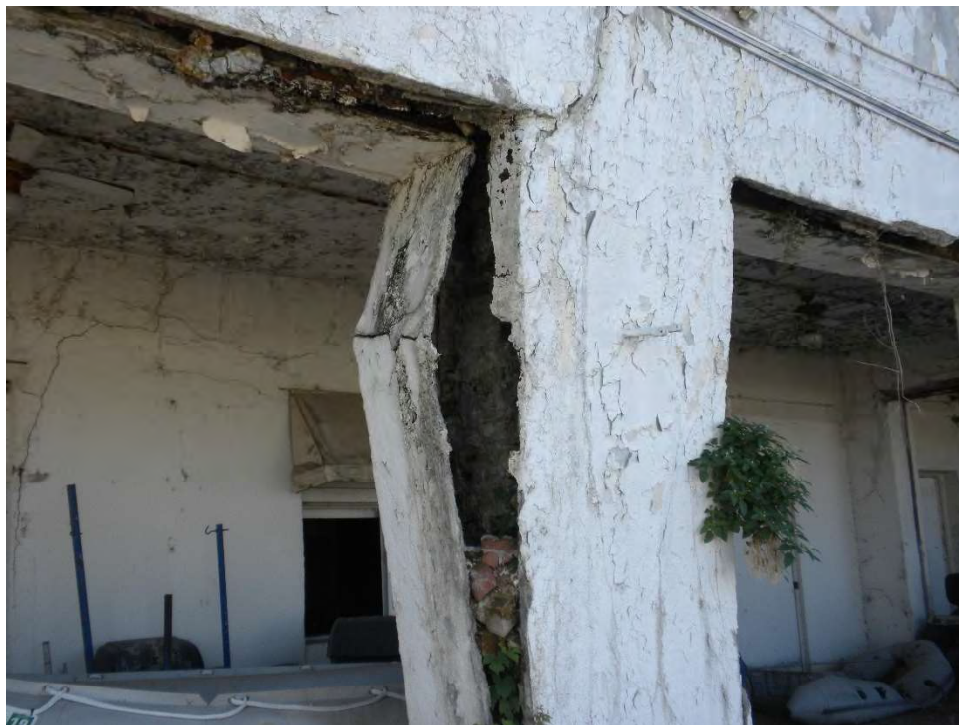
Photo 12 Debonded Stucco (Exterior Façade)
