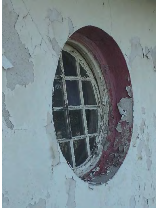
Photo 41 Weathered Condition Impeding Operation
