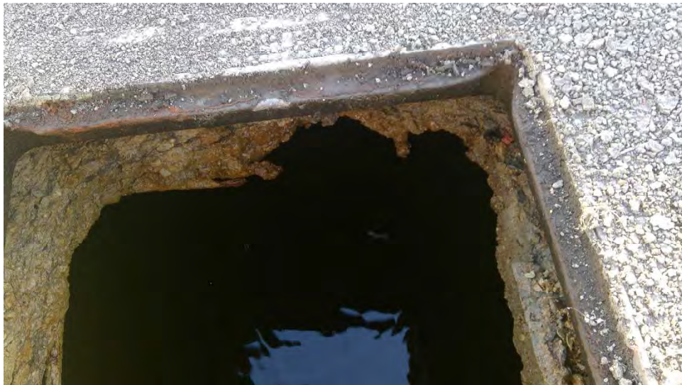
Photo 80 Deterioration Below Hatch
