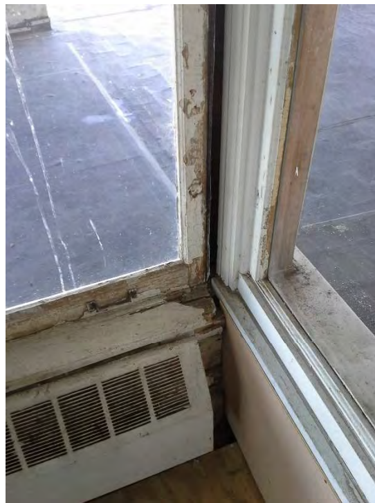
Photo 40 Splitting Wood Sill
