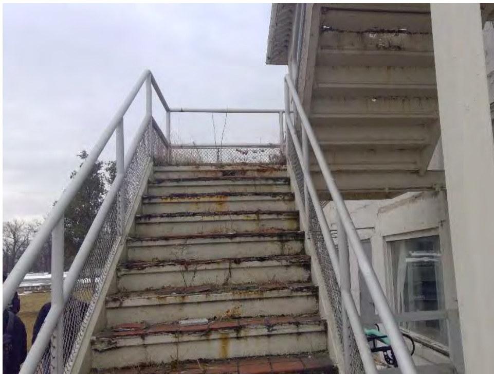
Photo 28 Northeast Staircase Corroded Steel
