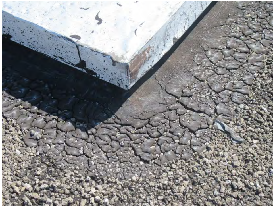
Photo 56 Damaged Flashing
