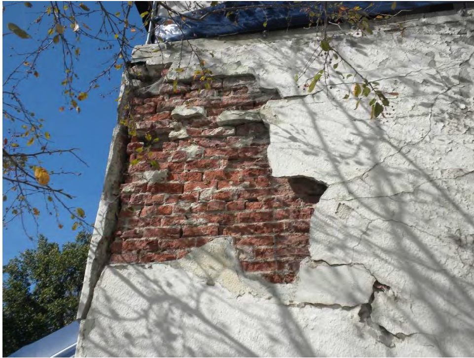
Photo 5 Damaged/Deteriorated Brick
