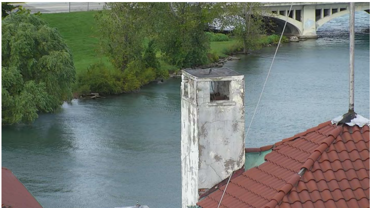
Photo 30 Scaled Stucco on Chimney
