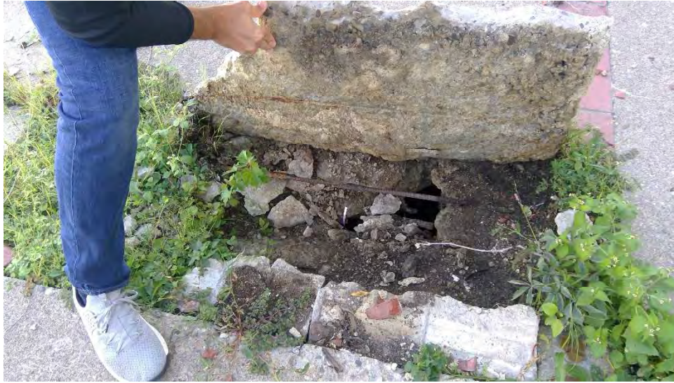
Photo 81 Hole Below Spalled Concrete
