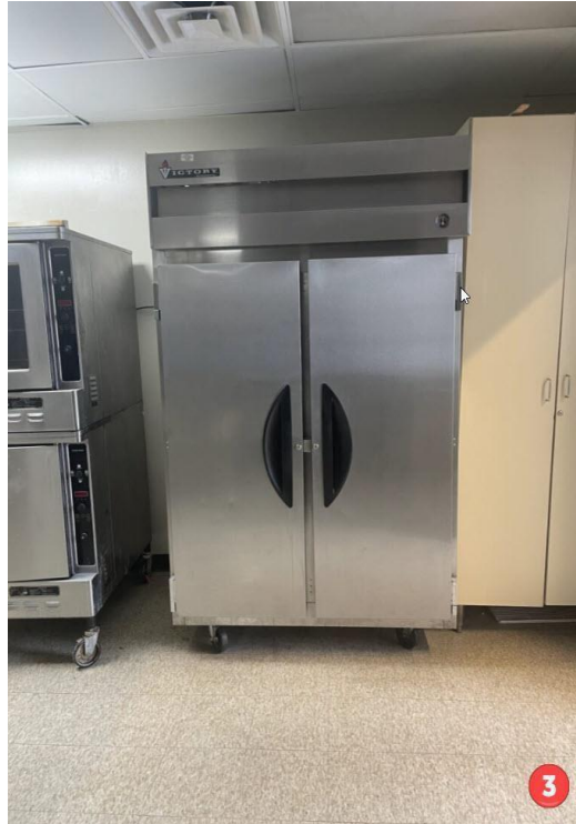
Figure 3. Double stack Convection Oven, Solid Door Roll-In Freezer, and Two Door Tall Cabinet (Left to Right)
