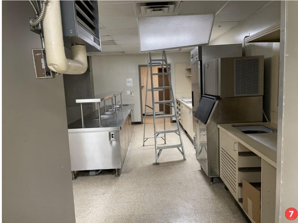
Figure 7. Food Preparation. Another view of steam table, ice machine, one-door refrigerator. Current work on electrical.
