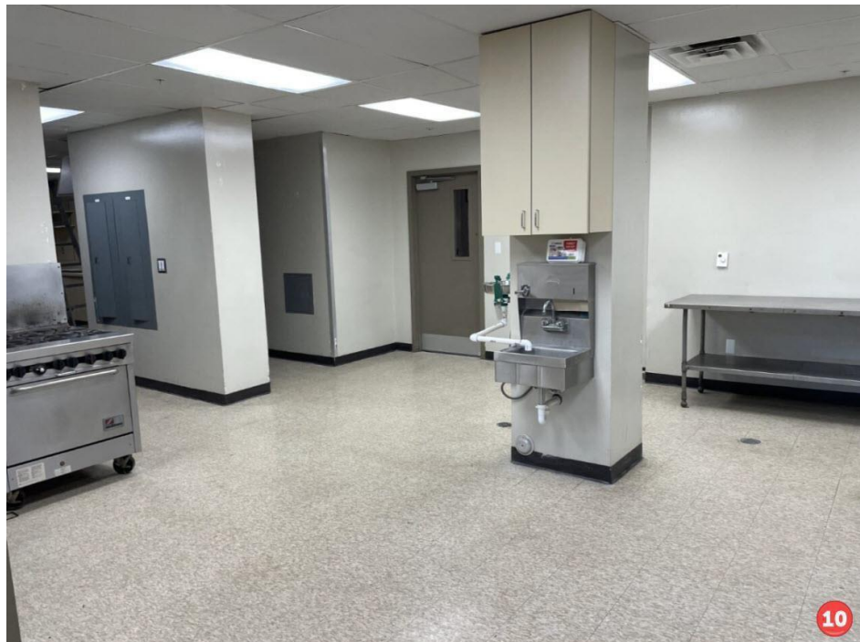
Figure 10. Alternative view of cleaning/washing station and storage/receiving section. Emergency eyewash and hand washing station.
