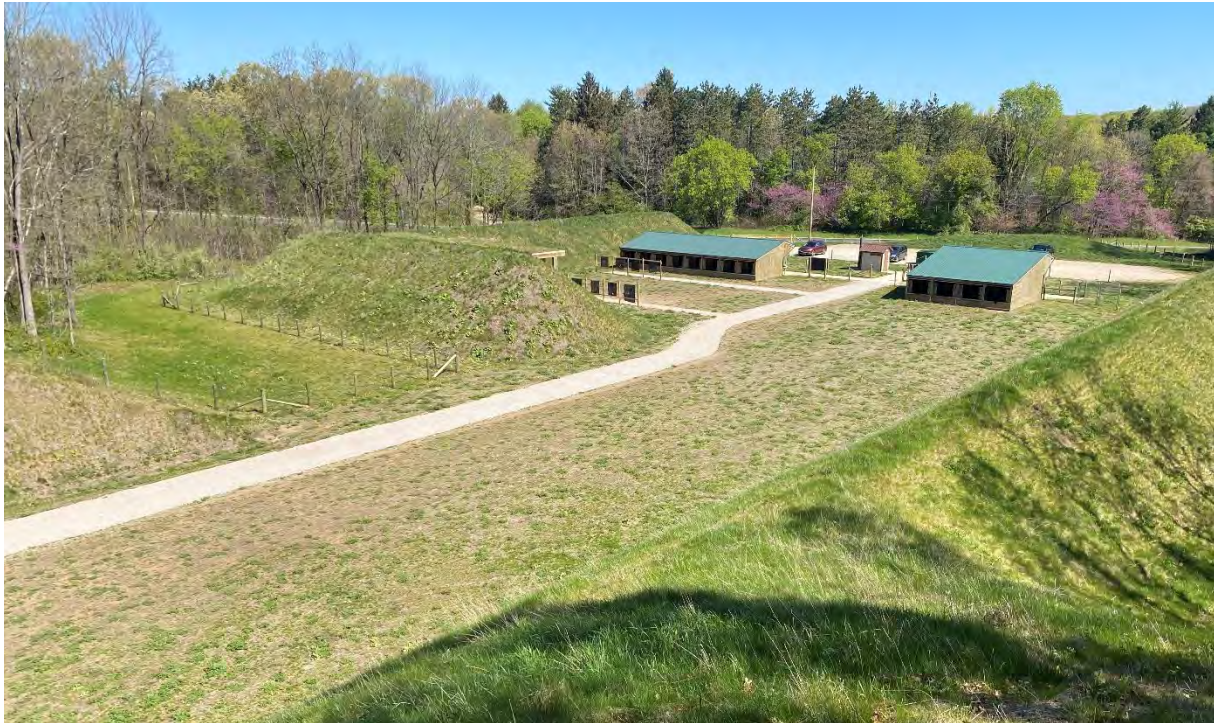
Figure 8. Photograph of the 15 ft. tall berms on the sides of the range and behind the targets of the pistol range and the 4 bay rifle shooting shed on the right and the 8 bay pistol shooting shed on the left.
