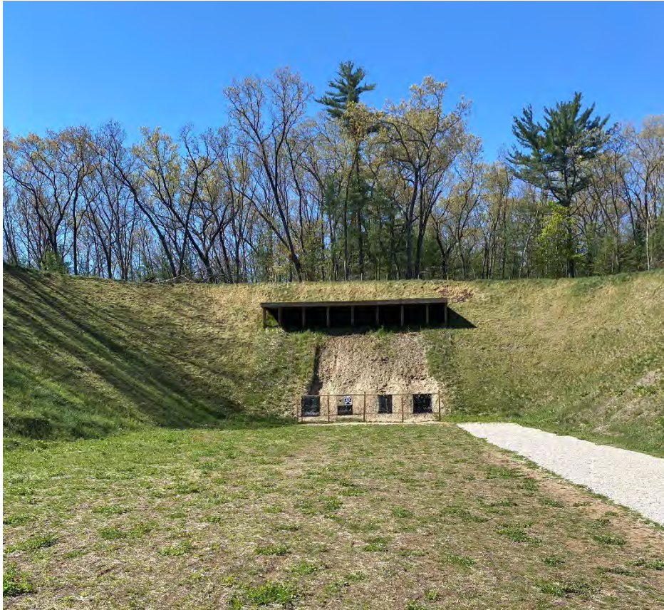
Figure 10. Photograph of the rifle range showing the berms on the sides of the range and behind the targets as well as the ricochet baffle above the targets.
