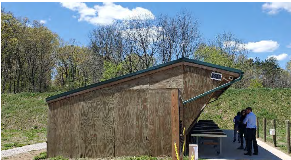
Figure 9. Photograph of the side of the pistol shooting shed. The walls of the shed are constructed of plywood on wood framing. The roof is a metal roof on plywood. The interior wall and roof surfaces of some of the bays are lined with sound absorbent glass fiber batts. The roof overhangs the shooting position. The shooters can sit or stand at the tables and their firearms are under the roof structure and within the walls of the shed when they fire. The depth of the shed in the direction of fire is 24 ft. 2 inches.
