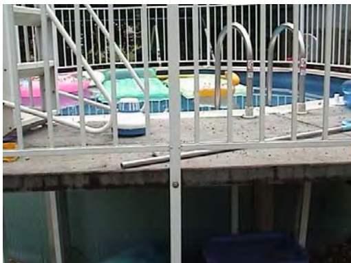
Figure 4c. Explosion/fire-associated debris (grit-like material) on pool decking, Romulus, Michigan (8/12/05). (EPA contractor photo.)
