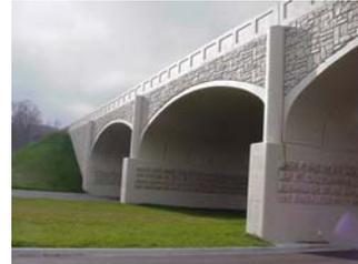
Sometimes using a CSS approach introduces new ways of constructing transportation projects. How such new practices are introduced should be part of the CSS process. For example, when this project was constructed, the use of concrete form liners was relatively new. Should a project's specifications require that a contractor be certified in using the new practice before they are allowed to bid on the project? How do we introduce new practices but still keep bidding competitive?
