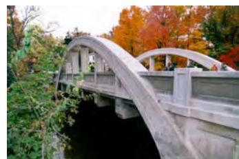
Merrick Street Bridge, Adrian, MI
