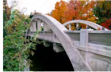
Merrick Street Bridge, Adrian, MI
