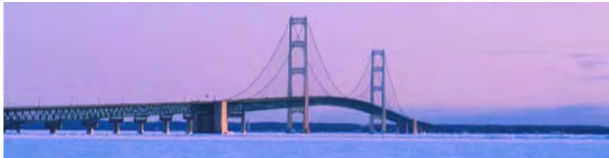
Mackinac Bridge, MI
