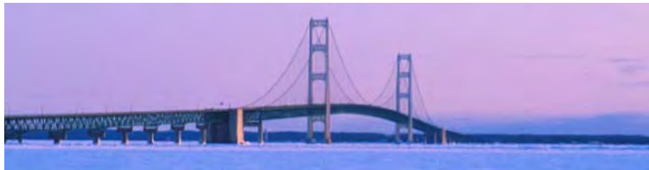
Mackinac Bridge, MI
