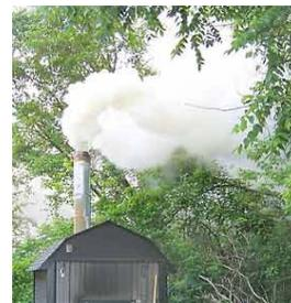
Most outdoor wood boilers create more pollution than a wood stove because they are designed to burn wood at lower combustion temperatures.
