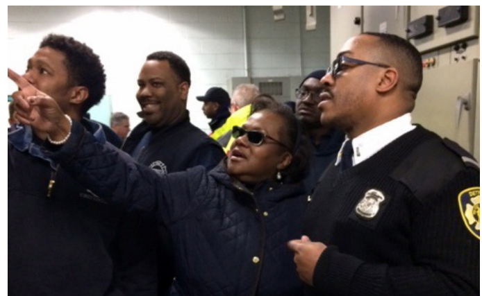
Inspector Elvira Chapman and Fire Department Lt. E. Davis discuss the facility generator during the familiarization tour.
