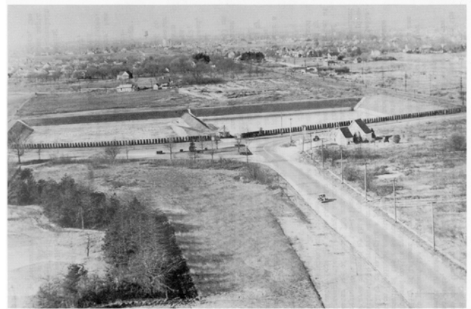
Figure 43. Photograph showing Rockaway Road recharge basin, Garden City, New York. (Courtesy of Department of Public Works, Nassau County, New York.)
