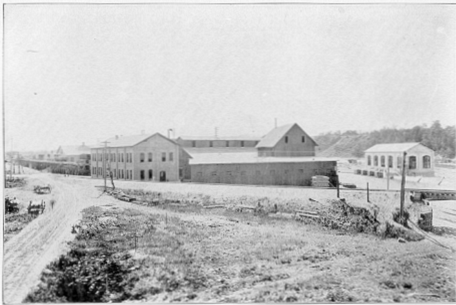
Plate XXII. General view Newaygo Portland Cement Co's plant.
