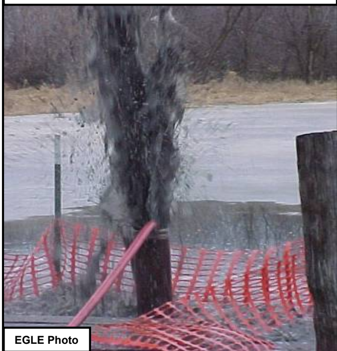
Surging sediment and debris out of an abandoned water well in Jackson County, Michigan
