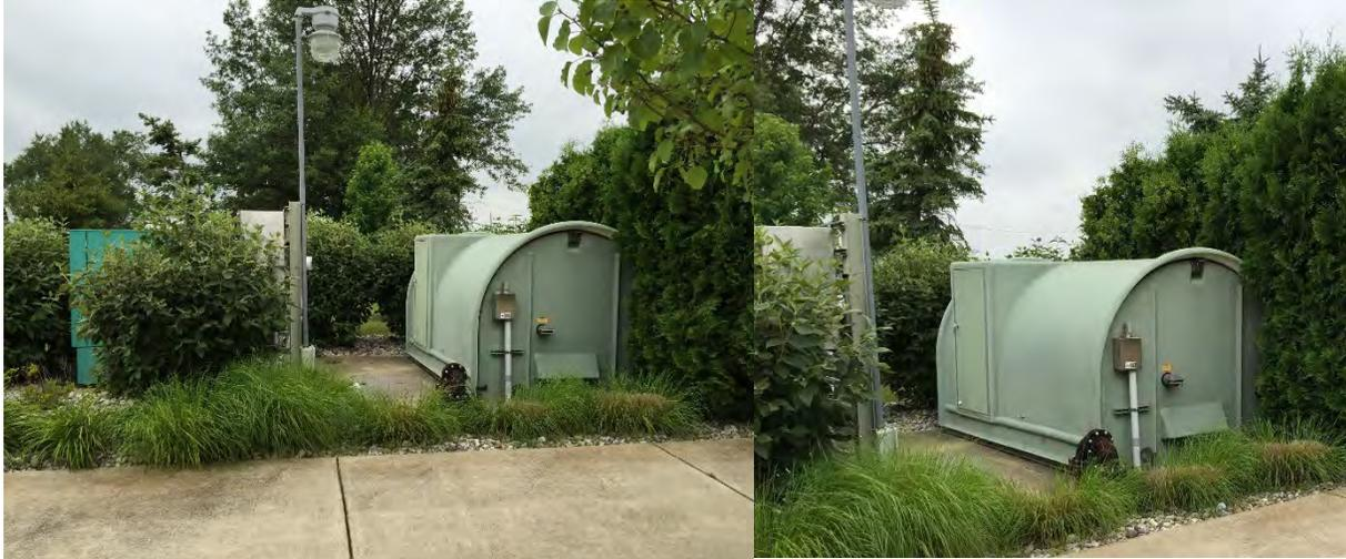
**Description:** Pump Station PS-7 is a duplex submersible pump station with an above ground fiberglass valve and control enclosure. The station serves a small residential development on the southwest corner of the Village. The station was originally constructed in 2003 and currently discharges to manhole 4-30, adjacent to the station via 4 inch plastic force main. The pumps and valves are in good condition. The controls and control cabinet are in good condition.
