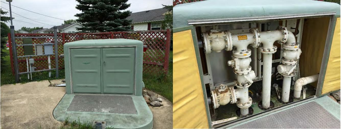
**Description:** Pump Station PS-5 is a duplex submersible pump station with an above ground fiberglass valve and control enclosure. The station serves a handful of properties on Oak Street south of Roosevelt Street. The station was originally constructed in 1999 and currently discharges to manhole 3-59 in Oak Street north of Country Heritage via 4 inch plastic force main. The pumps and valves are in good condition. The controls and control cabinet are in good condition.
