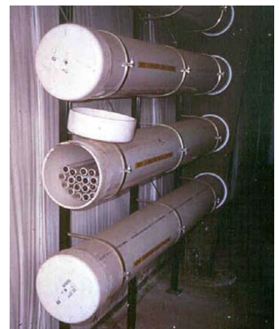
Example of one type of universal waste storage. End cap removed for taking picture.
