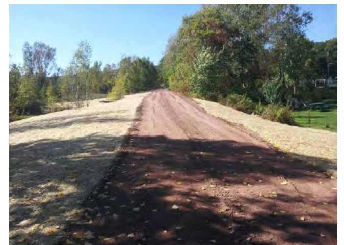
Photo 4: Placement of seed, straw mulch blankets, and SESC BMPs installation. Photo taken on 9/27/15.
