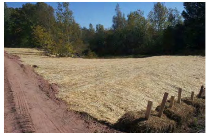
Photo 2: Placement of geotextile separator fabric (demarcation layer) over area. Photo taken on 9/25/15.
