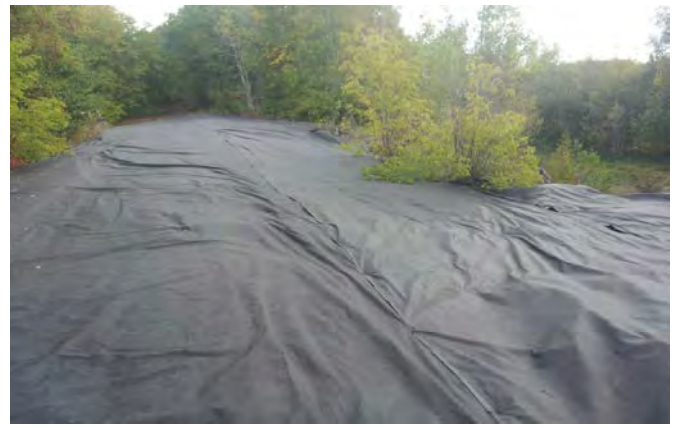
Photo 2: Placement of geotextile separator fabric (demarcation layer) over area. Photo taken on 9/25/15.
