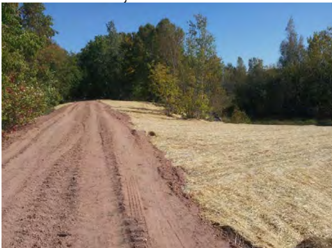
Photo 5: Placement of 1-foot thick layer of gravel over the trail surface. Photo taken on 9/27/2015.
