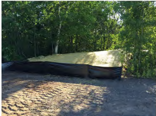
Photo 5: Installation of SESC best management practices. Photo taken on 7/13/2016.
