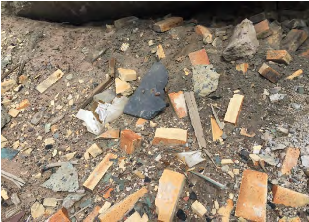
Photo 3: ACBM prior to removal at Mineral Building. Photo taken on 8/10/16.
