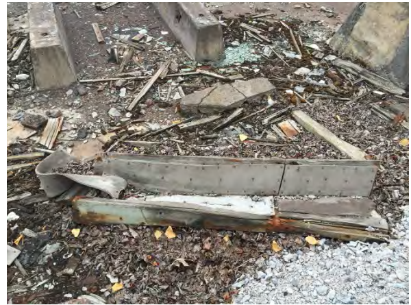
Photo 2: ACBM prior to removal at Tamarack Processing Area. Photo taken on 8/20/16.
