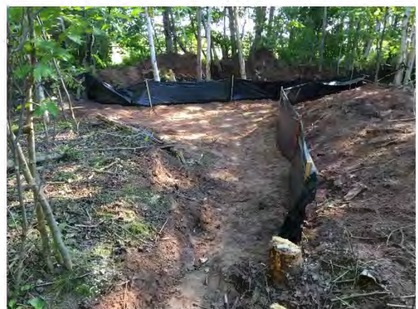
Photo 6: Confluence with north ditch after clean out. Photo taken on 8/25/16.
