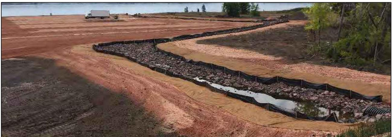
Photo 10: View looking southeast to the installation of the coconut shell erosion control blanket along the ditch. Photo taken August 14, 2017.
