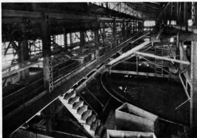
Figure 1. 40 ft. thickeners in north flotation plant, Lake Linden.
