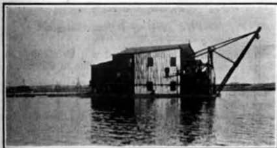
Dredge and portion of pontoon line
