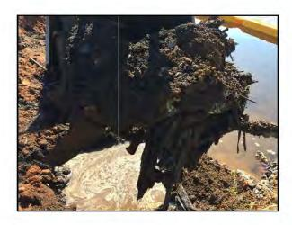
Photo 8: View of white sludge material mixed with sediment, excavated from shoreline as part of Container #10. Photo taken July 11, 2017.
