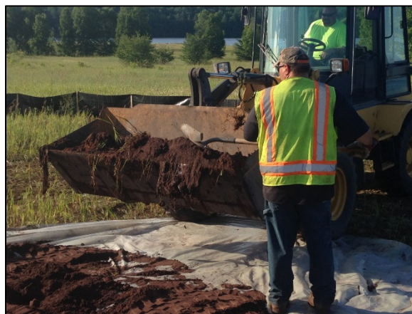
Photo 8: View of plastic drum liner and seep material during excavation of Seep #2. Photo taken on July 13, 2017.
