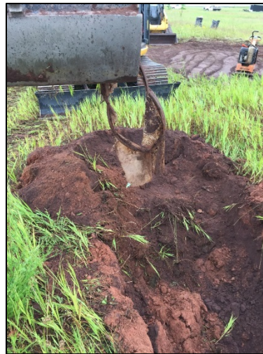
Photo 8: View of plastic drum liner and seep material during excavation of Seep #2. Photo taken on July 13, 2017.
