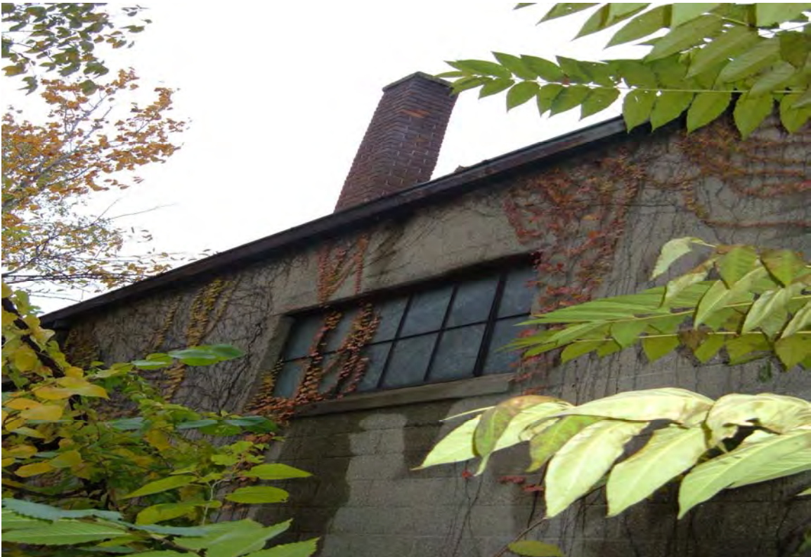
Photograph 2: View of remaining stack on southwest side of building.
