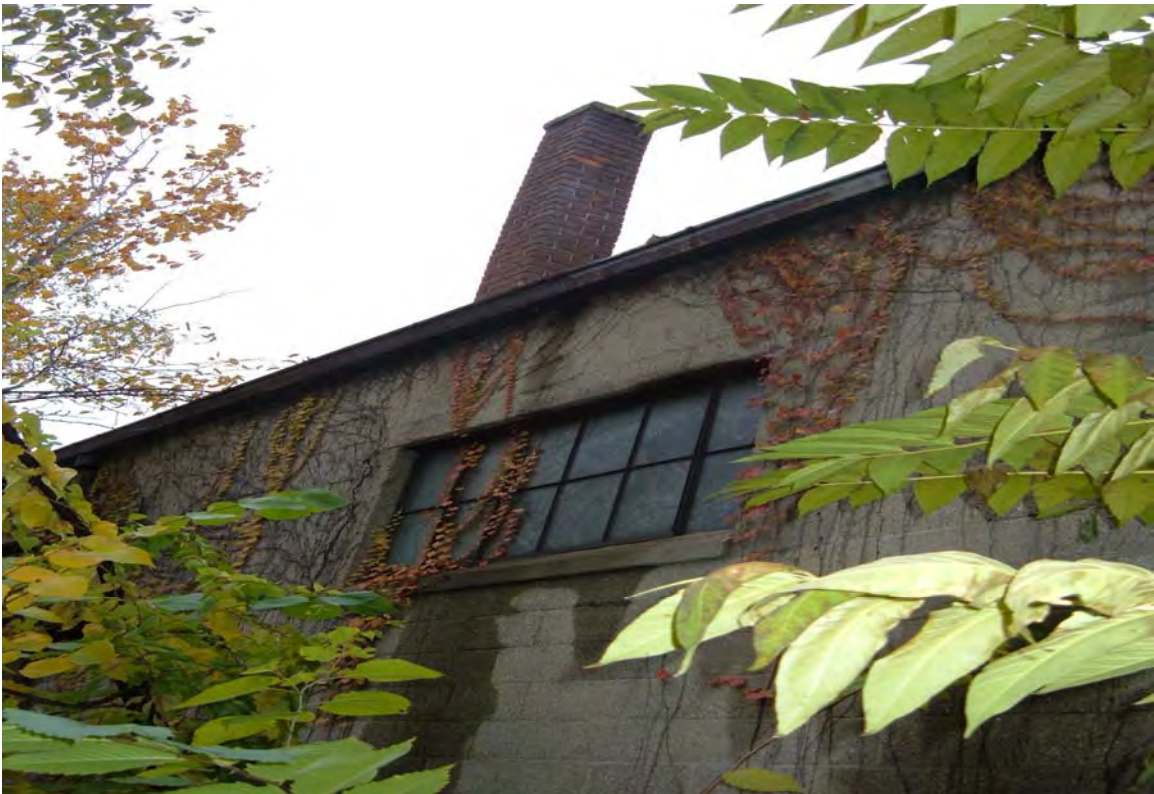
Photograph 2: 10/27/06: View of remaining stack on southwest side of building.
