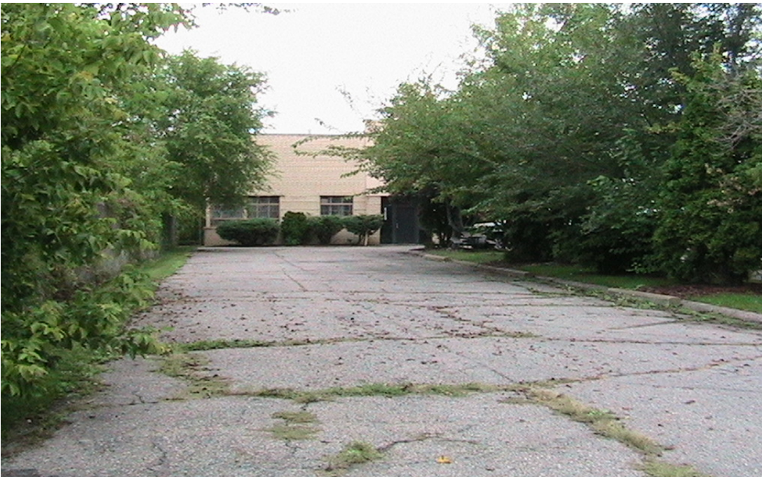
Photograph 2: View of northwest side of the existing building from Mt. Elliot. Location of MTE19430-01 through 03 (in central boulevard portion) and MTE19430-04 and 05 (along fence line.).
