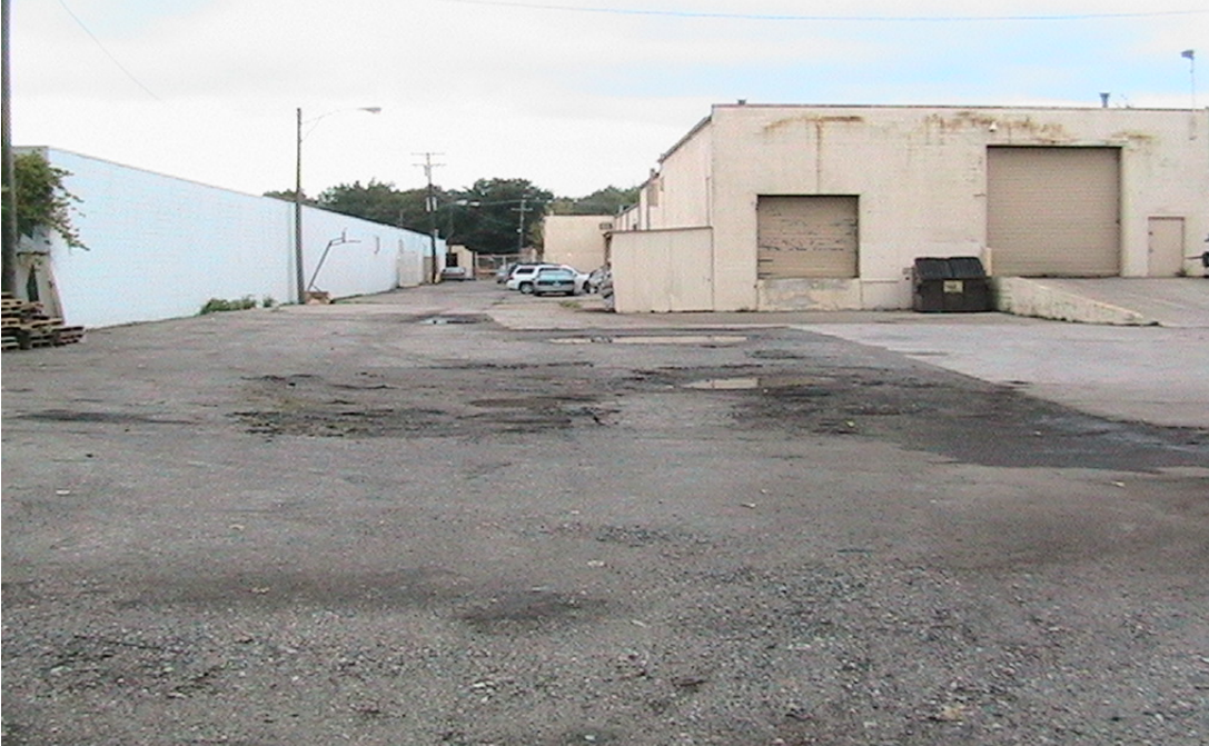
Photograph 1: View of east side (back) of existing building. Exposed ground surface is present along the northeast side of the building. WESTON attempted to collect a sample in this area, but could not collect sufficient sample material.
