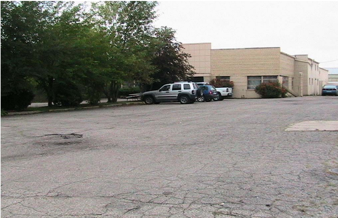
Photograph 3: View of southwest side of the existing building from Mt. Elliot.
