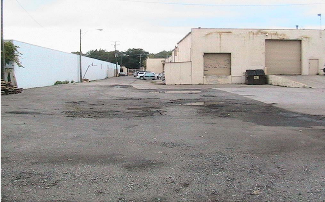
Photograph 1: View of east side (back) of existing building. Exposed ground surface is present along the northeast side of the building.
