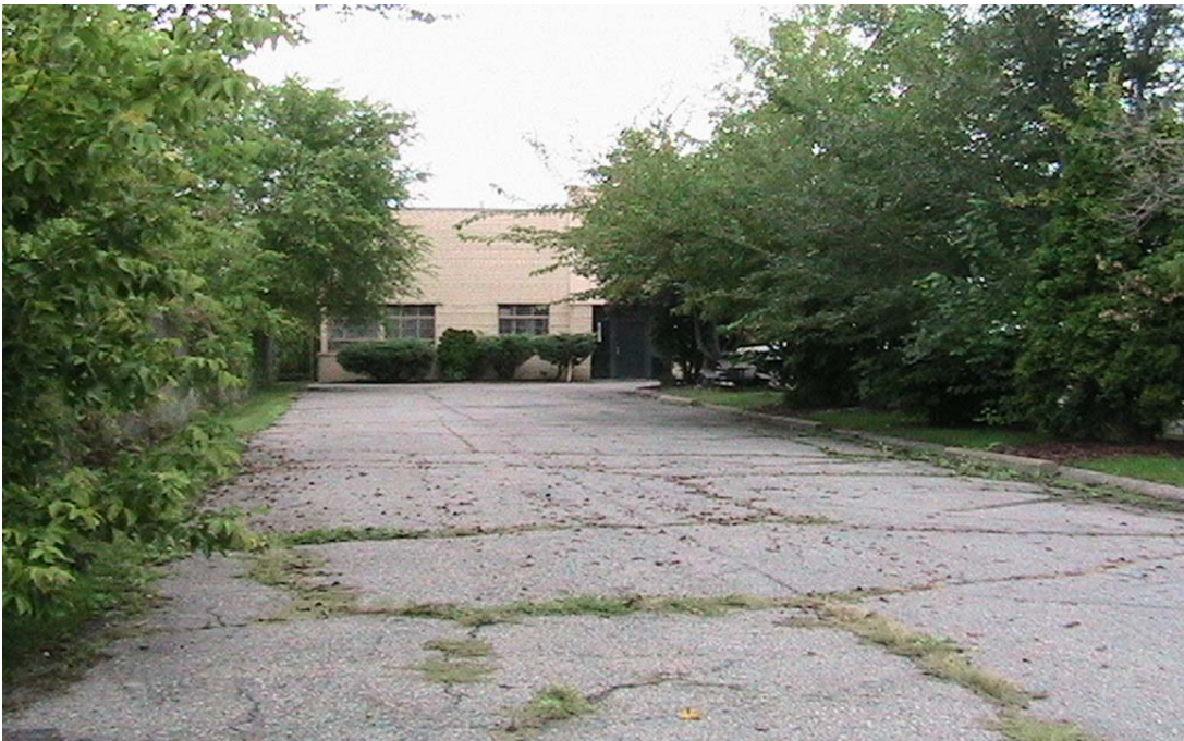
Photograph 2: View of northwest side of the existing building from Mt. Elliot. Note the location of green spaces on the north and central (boulevard) portions of the parking lot.
