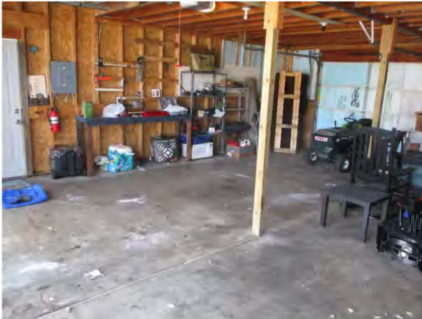
Exhibit 3. Attached Garage at 34367 Capitol Street
