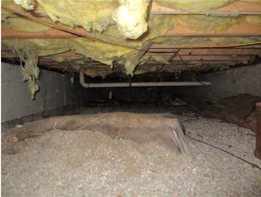
Exhibit 2. Crawlspace at 12017 Brewster Street
