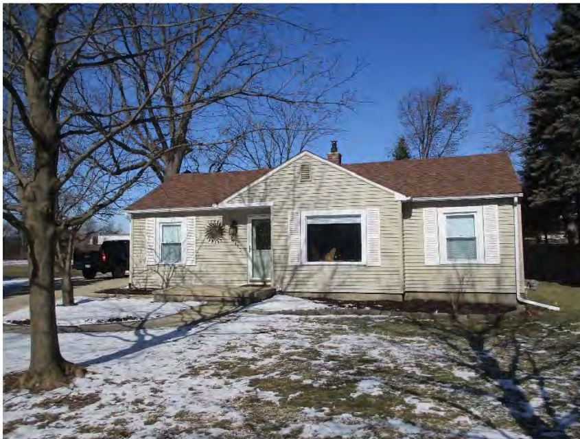
Exhibit 1. Front view of the residence at 34480 Capitol Street
