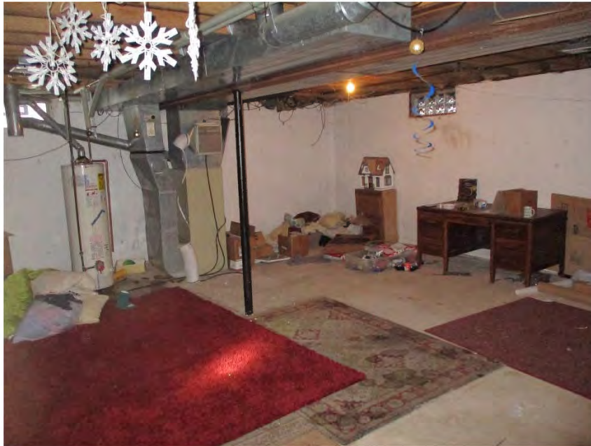
Exhibit 2. Basement at 34940 Beacon Street
