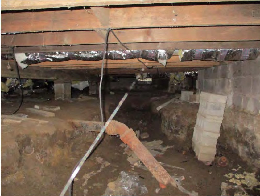
Exhibit 2. Crawlspace at 34591 Beacon Street
