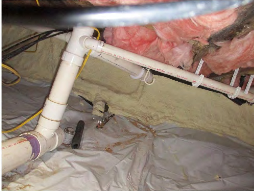
Exhibit 2. Crawlspace at 34682 Beacon Street
