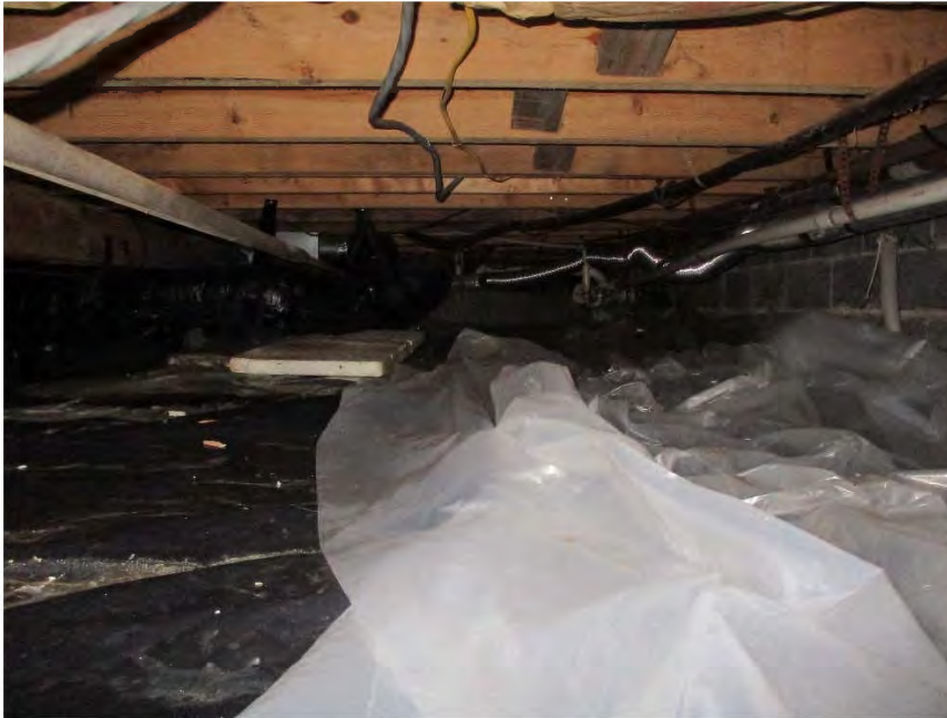
Exhibit 2. Crawlspace at 34880 Capitol Street.
