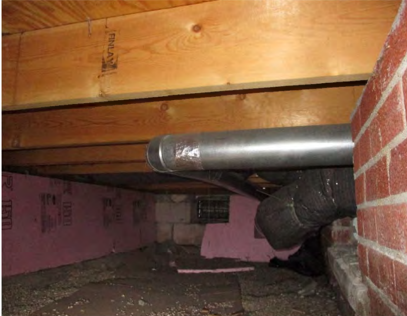
Exhibit 2. Crawlspace at 34990 Beacon Street
