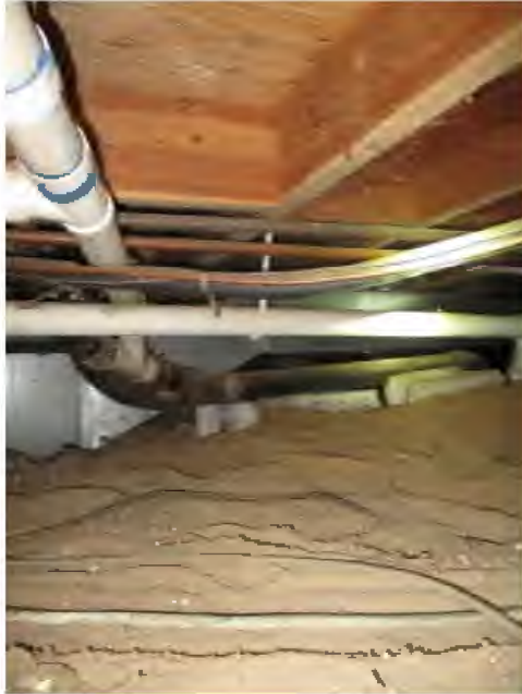
Exhibit 2. Crawlspace at 34367 Capitol Street.
