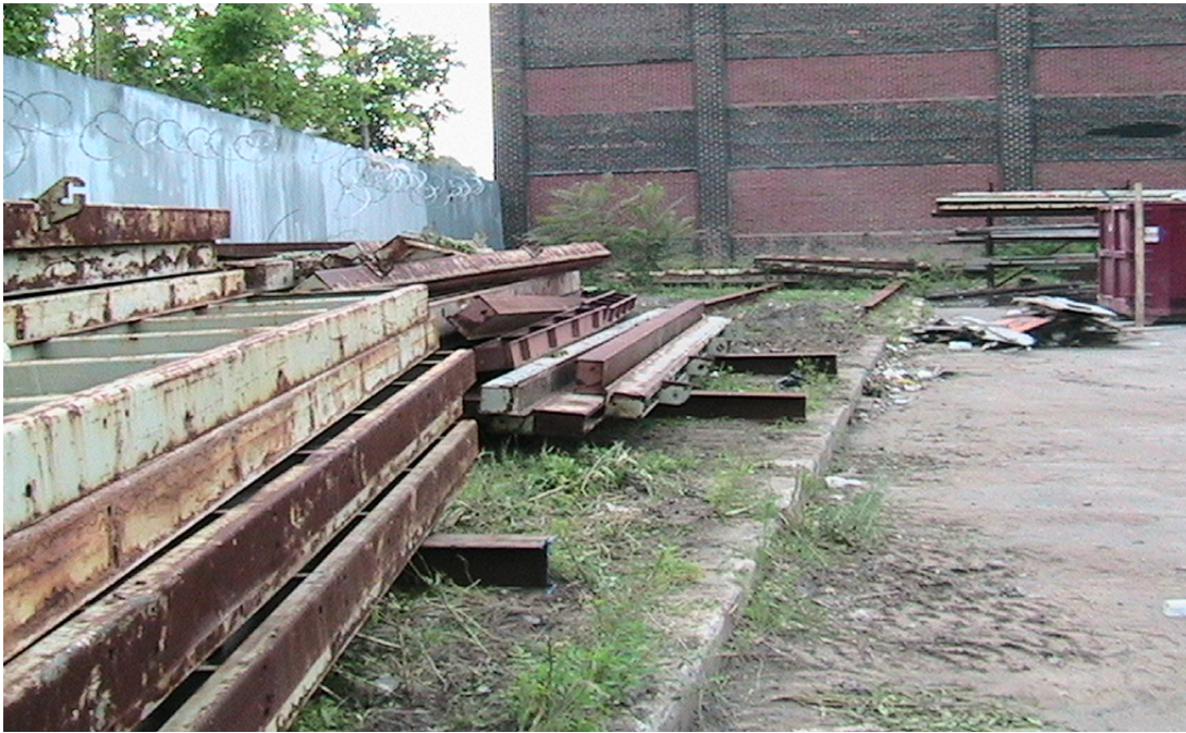
Photograph 3: Northeastern side of the property facing south.
