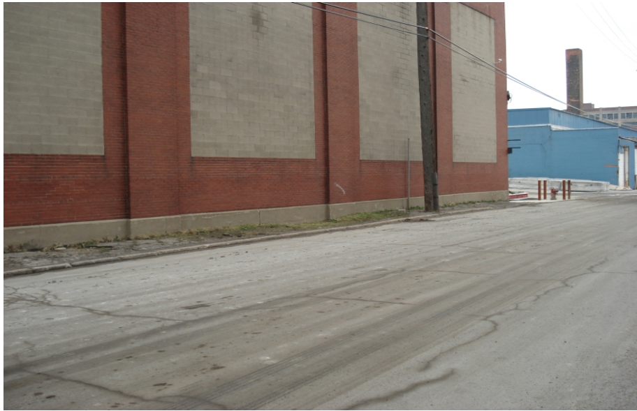
Photograph 1: Facing southeast along the west side of Stress Con on Hartwick Ave. – location of samples EEU-1640-05 through EEU-1640-06.
