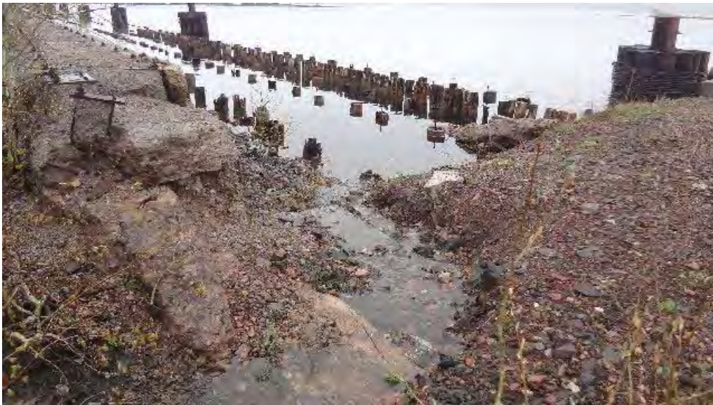
Photograph 36: 5/12/15: View looking northeast at collected storm water at the former Coal Dock property discharging to Torch Lake through eroded channels along the bulkhead. Photograph taken by D. Liebau.
