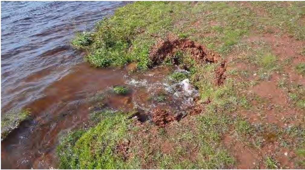
Photograph 25: 10/06/14: View looking down/south at cap erosion along the shoreline in the Lake Linden Recreation Area. Photograph taken by D. Liebau.
