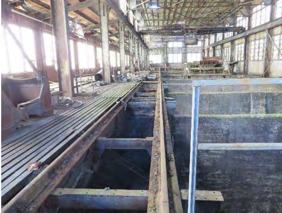
Photograph 19: 7/16/14: View looking south at the interior of the former Mineral Building. Mineral storage bins, more than 20 feet deep, are shown along the right side of the photograph.. Photograph taken by A. Keranen.
