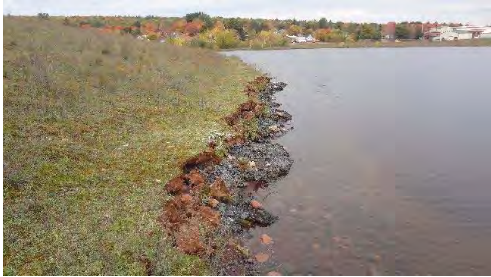
Photograph 31: 10/07/14: View looking northwest at exposed slag in the Hubbell Beach and Slag Dump Area. Elevated lake levels have resulted in the erosion of cap material along the shoreline of Torch Lake. Photograph taken by D. Liebau.
