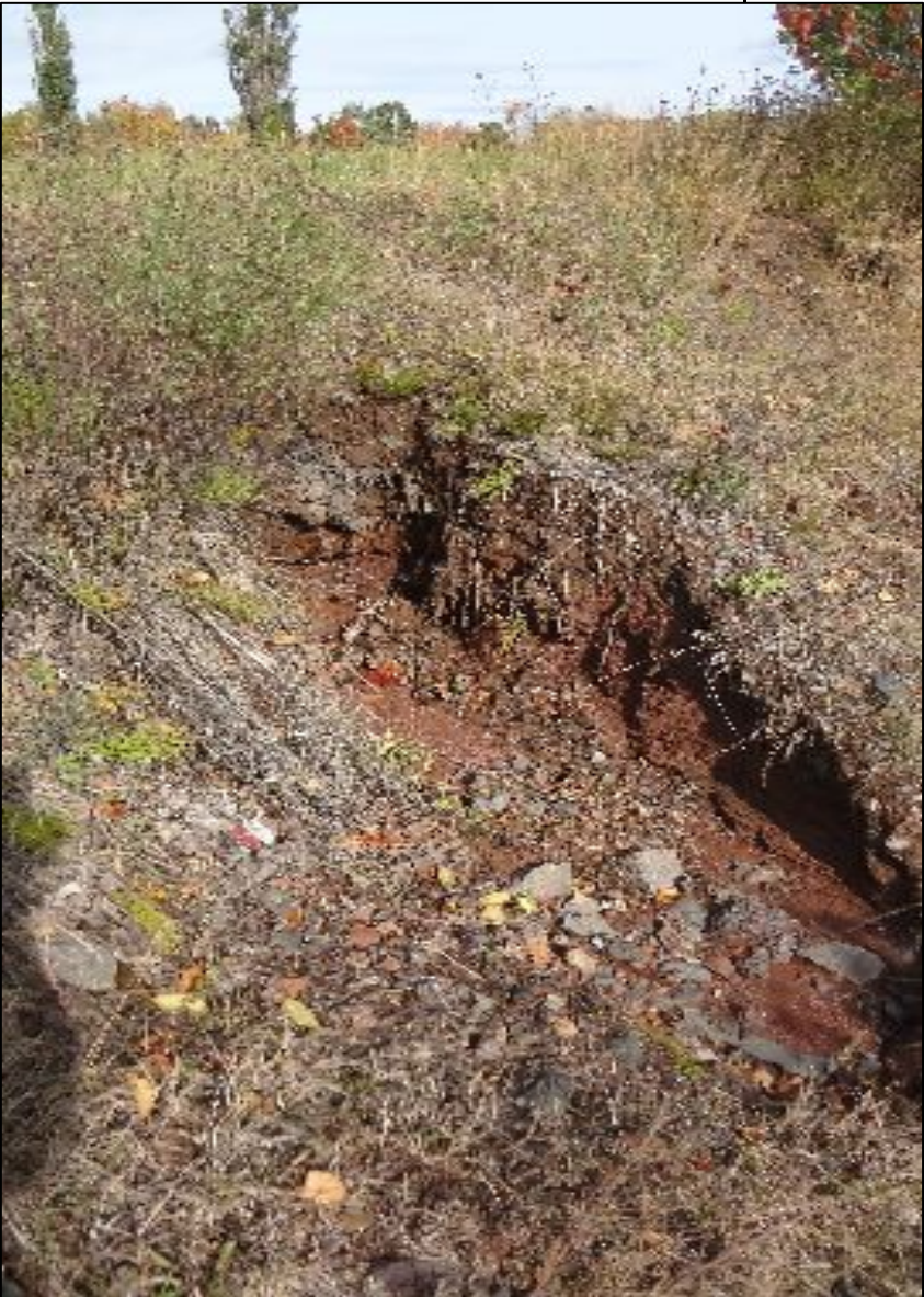
View looking west/northwest at an area of cap/shoreline erosion north of the marina.
