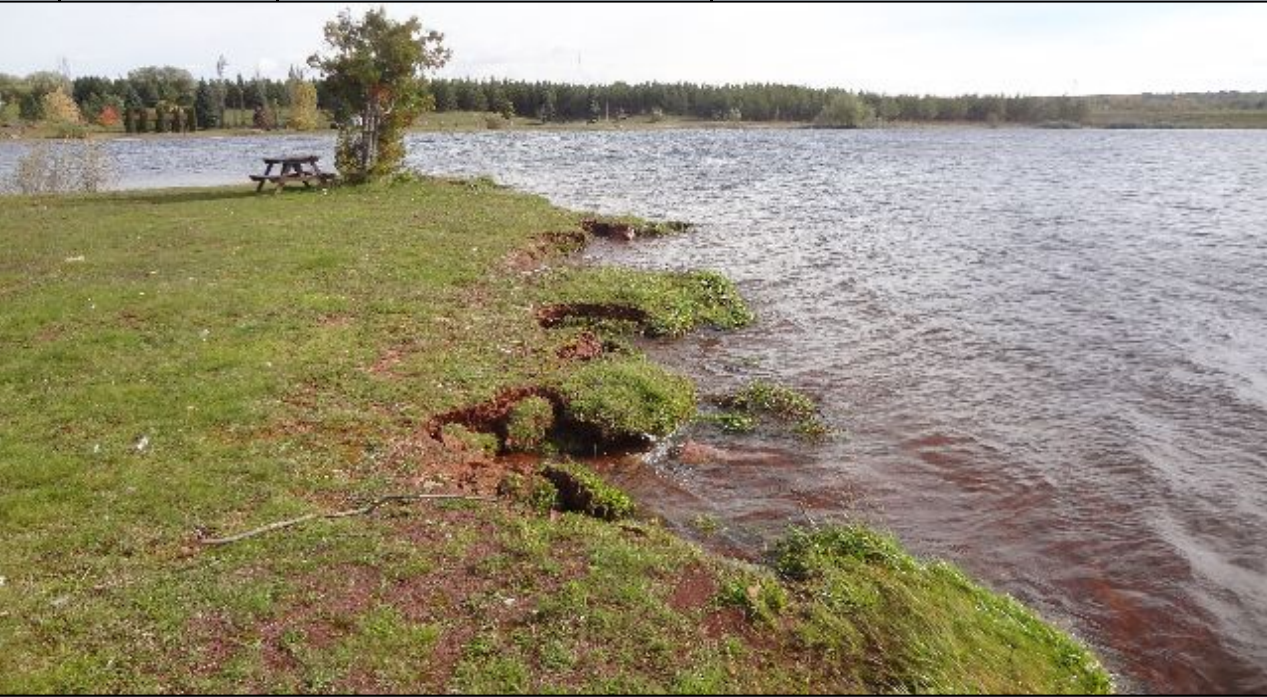
View looking east at eroded portions of the cap/shoreline in the eastern portion of the subject property.
