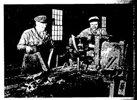
Stripping machine for recovering lead and copper from cable
