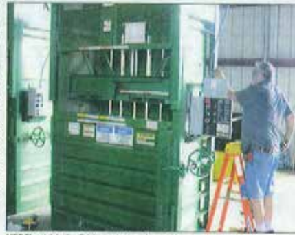
MKE Electric's Jim Fulshe works to get one of two new balers up and running at
