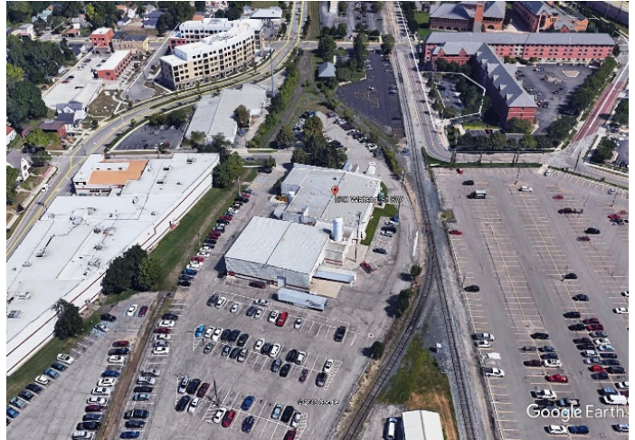
Viant Medical Facility
