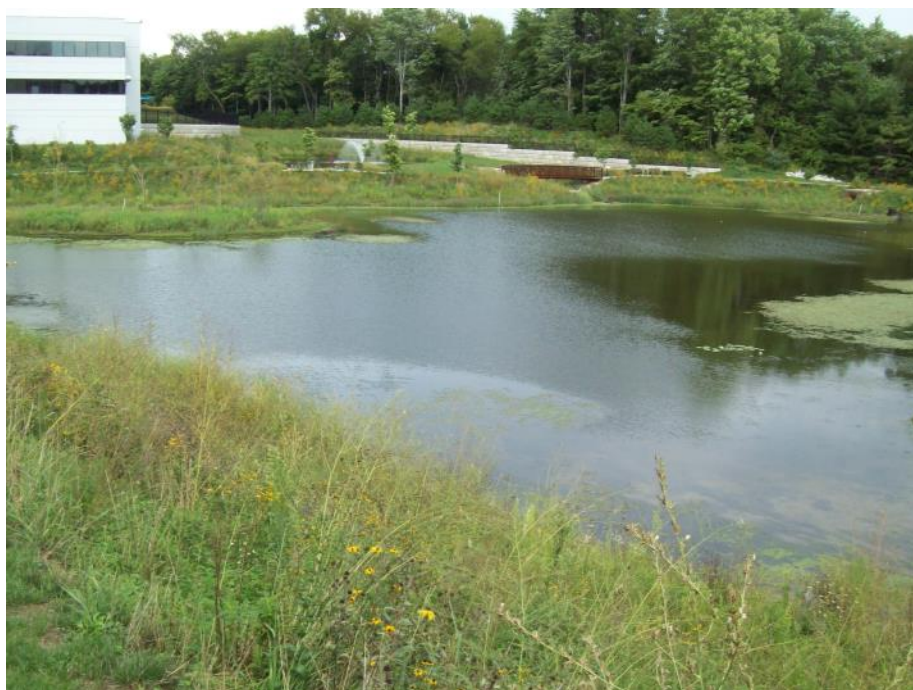
Pond Elevation lowered 5.5', Creates 50 ac/ft more storage
