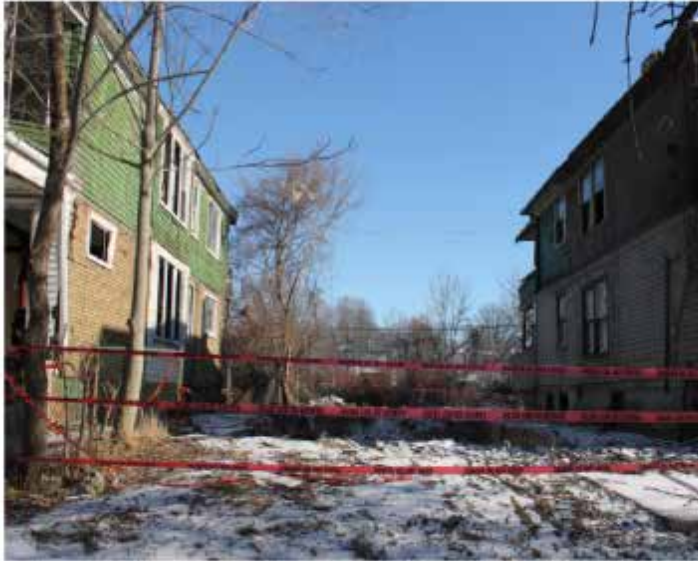
Demolition in progress
