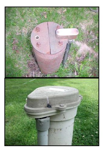
8. **Cross Connections with Contamination Sources** (such as an unapproved water supply tied in series with the well and stop and waste yard hydrants). Cross connections provide a means for the backflow or backsiphonage of contaminants into the water supply. Cross connections must be eliminated by installing approved cross connection control devices.
