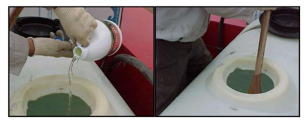
If calcium hypochlorite is used as the source of chlorine, it should be dissolved in a pail of water before being added to the prepared source water. After being added to the bulk tank and thoroughly mixed, the calcium carbonate impurities should be allowed to settle to the bottom of the tank. The clear solution above the sediment is then drawn off for discharge into the water well. Use sodium hypochlorite if the well water has more than 100 ppm dissolved calcium (calcium carbonate).
